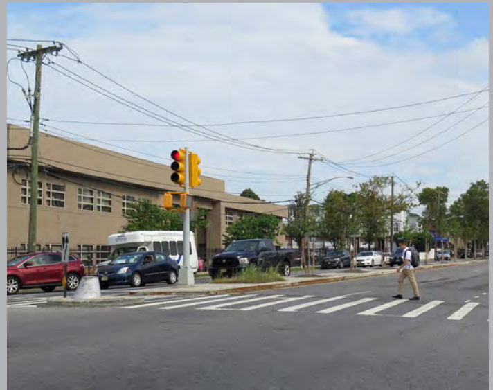
Richmond Avenue & Moroni Street, Staten Island, After
