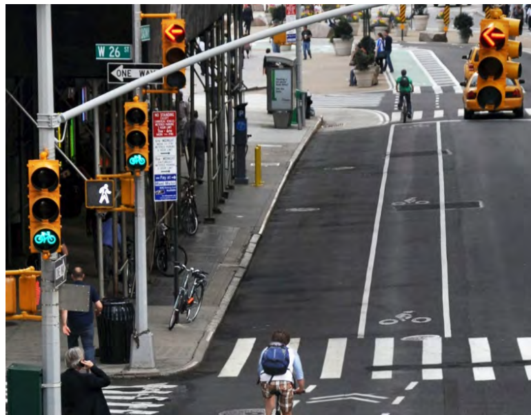
Turning Safety Signal Treatment: Broadway & 26 Street, Manhattan
