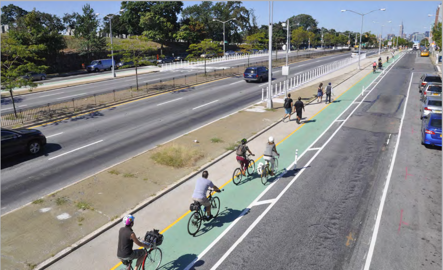
Queens Boulevard & 55 Street, Queens, After
