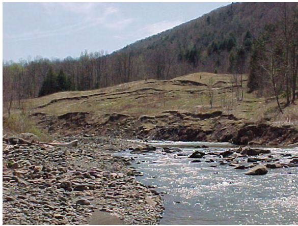
Figure 4.12. Large failing bank at Conine prior to restoration.
