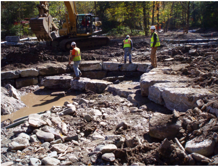
Figure 4.10. Double cross-vane during construction at Holliday Brook.
