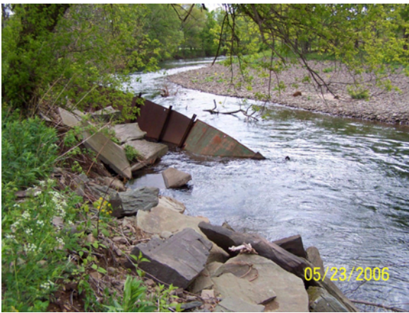
Figure 4.16 Margaretville demonstration restoration project site pre-construction.
