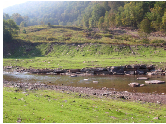
Figure 4.13. Large failing bank at Conine after restoration. The floodplain bench was added to relieve pressure on the slope.
