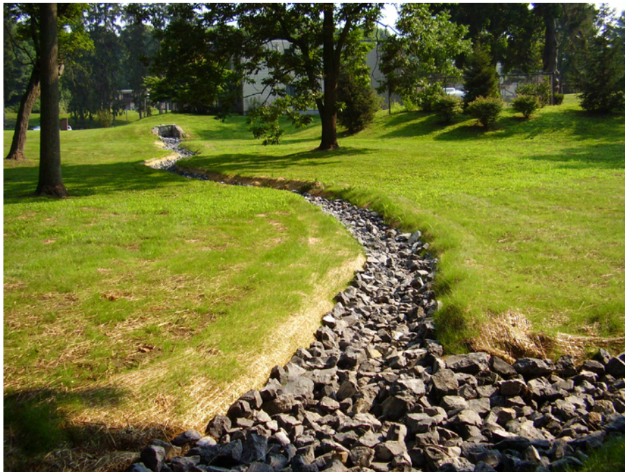
Figure 4.23. Swale repair at Vista on the Lake.
