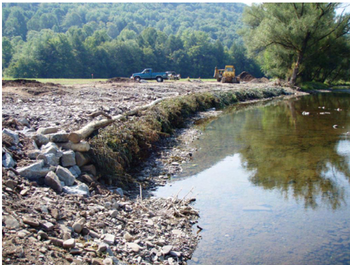
Figure 4.18. Live crib wall post-construction.
