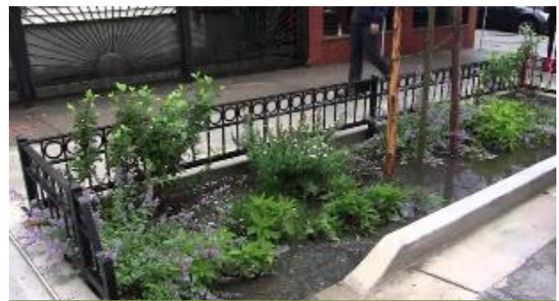
Curbside Rain Garden (Bioswale)
