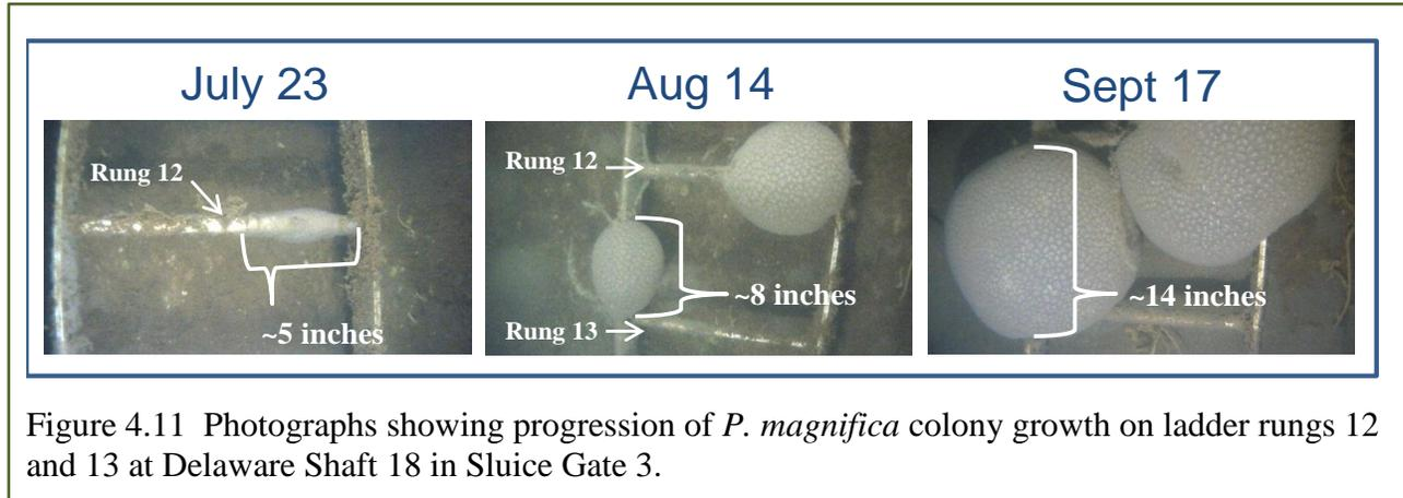
Figure 4.11 Photographs showing progression of *P. magnifica* colony growth on ladder rungs 12 and 13 at Delaware Shaft 18 in Sluice Gate 3.
