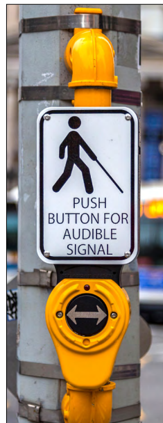
Above: A DOT employee installs an APS pushbutton. Right: A person who is blind uses an APS pushbutton before entering a crosswalk.
