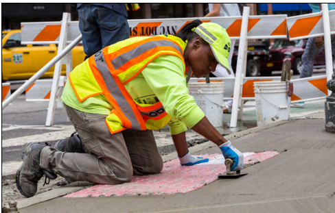
Above: A DOT employee installs a new pedestrian ramp. Right: A person in a wheelchair enters a sidewalk via a pedestrian ramp.
