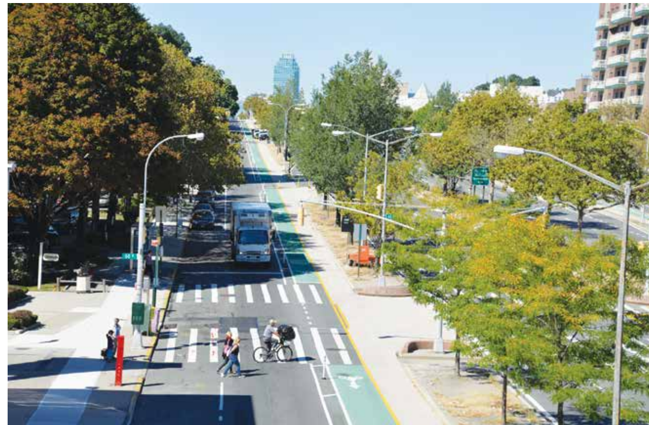
▲ As one of NYC DOT’s Vision Zero Great Streets, the agency has begun to add protected bike lanes, widened crosswalks, and extended medians.
