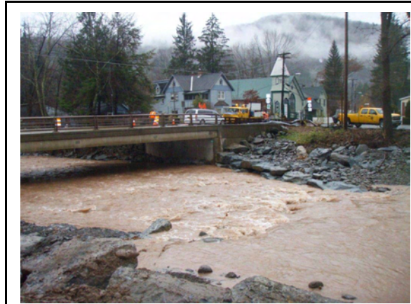
Figure 4.20 View of Stony Clove Creek at Phoenicia and Main Street bridge following post-flood response channel restoration work. Note cross vane extending upstream of bridge.
