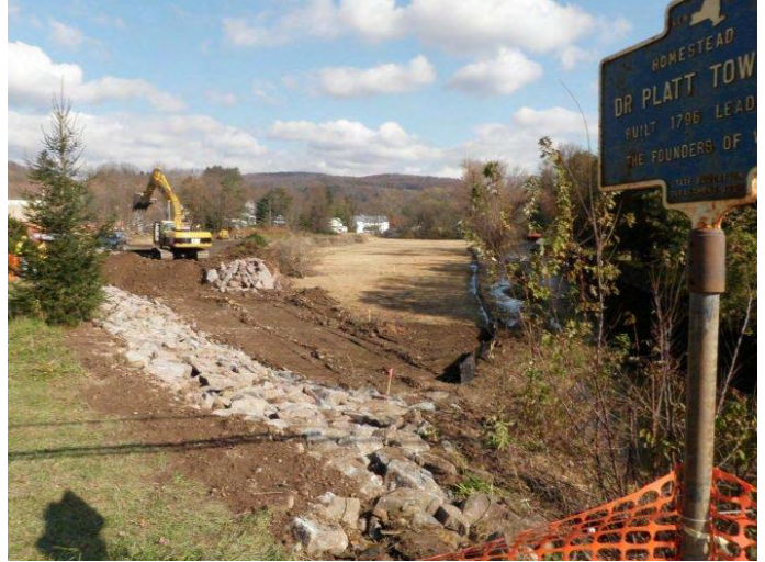
Figure 4.18 Fill removal at Village of Walton floodplain restoration.
