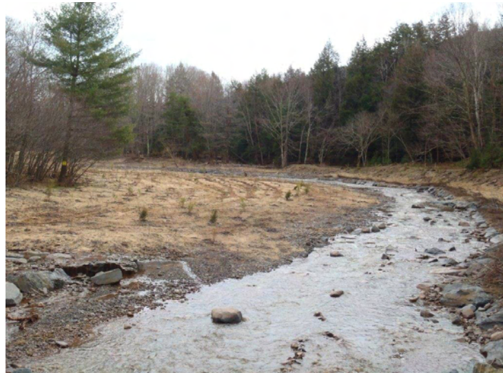
Figure 4.22 East Kill at Vista Ridge following restoration, with the stream back in its historical channel aligned with the bridge, the remainder of the site restored as wetland and floodplain, and the profile of Vista Ridge Road lowered to allow for flood flows.
