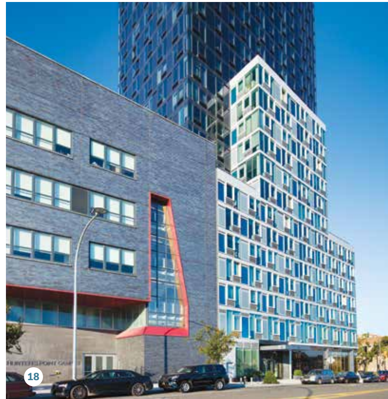
14. Windows and Doors: The SHoP-designed façade (visible here at the Crossing building) integrates HVAC units into window systems, incorporating the louver panels at the exterior, which streamlines the visual impact of the building system components.
