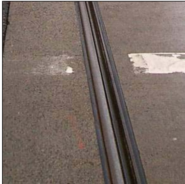
Figure 2-11: Flange Gap
