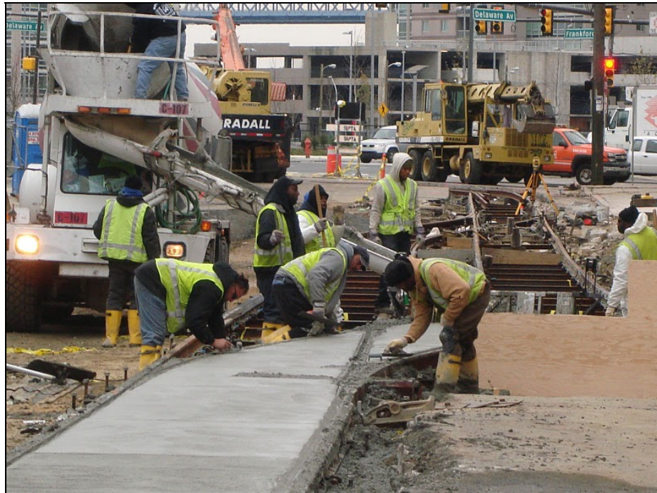
Figure 4-10: Route 15 Loop Construction along Frankford Avenue
