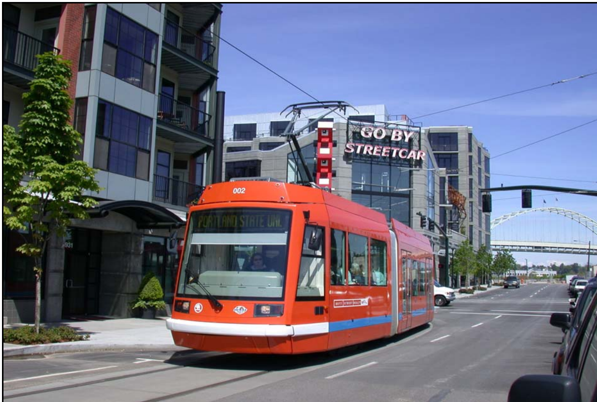
Figure 2-18: Portland Streetcar Overhead Contact System
