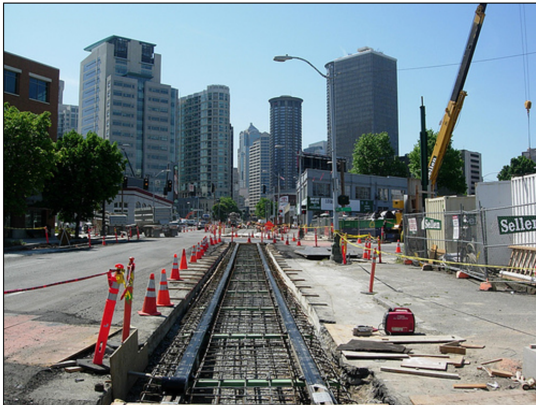
Figure 3-2: South Lake Union Streetcar Construction
