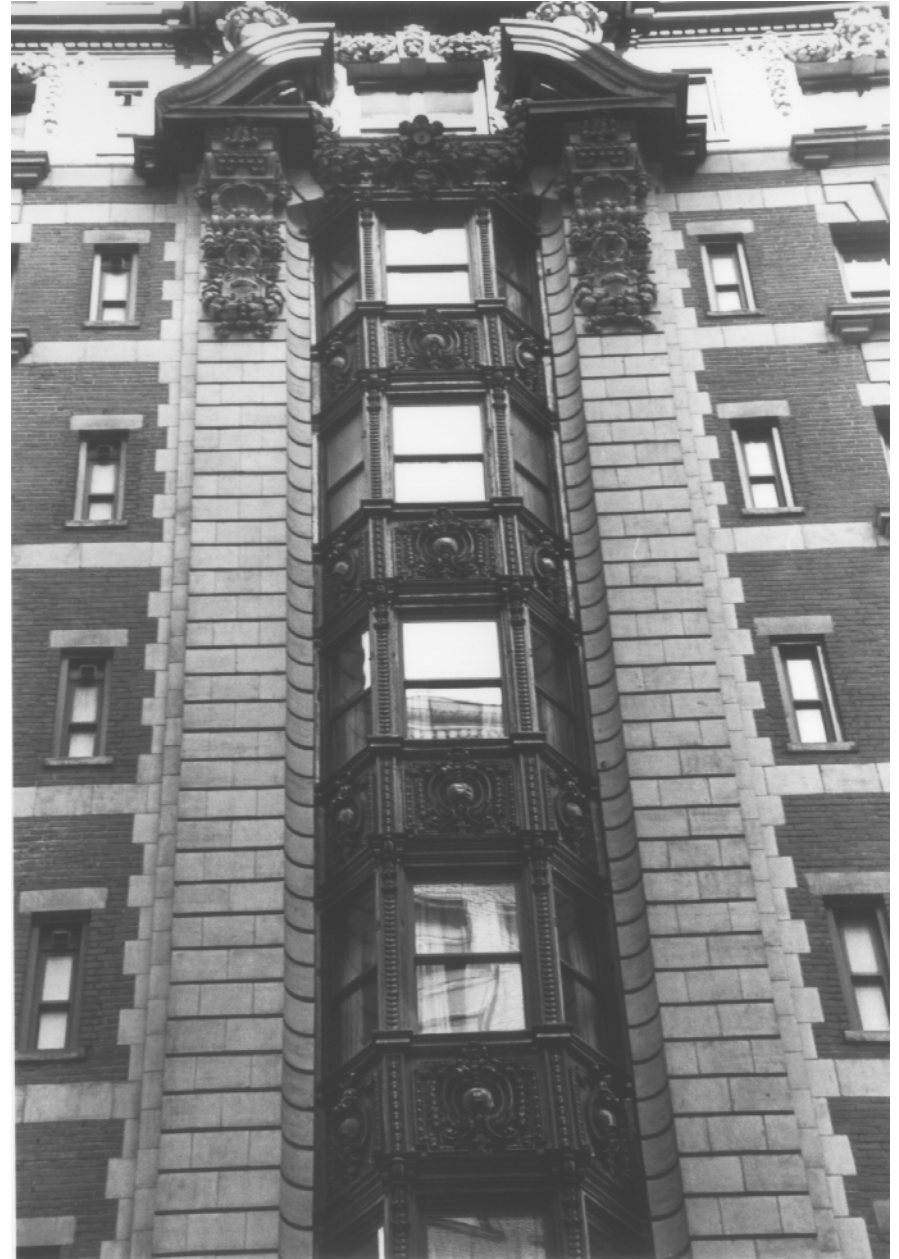
(Former) Aberdeen Hotel (now Best Western Manhattan Hotel), upper facade detail 17-21 West 32 nd Street, Manhattan
