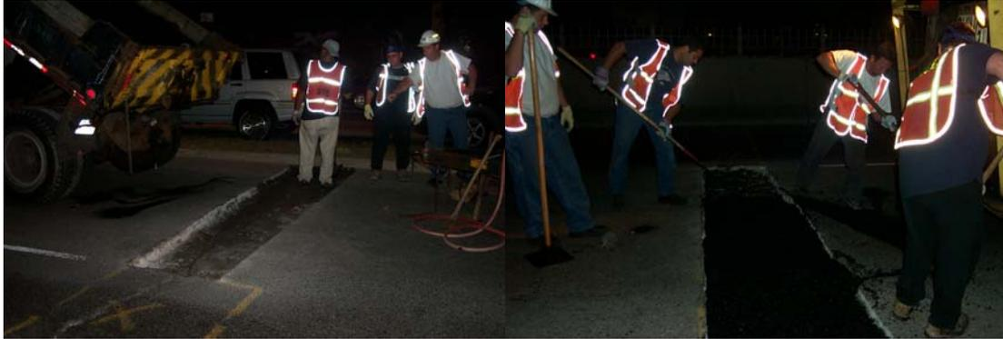
Break-Out and Removal of Old Asphalt at the Tillary Street Ramp to the Brooklyn Bridge
