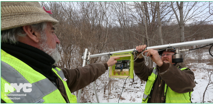
Glenn Horton, left, and Francis Huber work to install the radar device on a metal pole in the woods of Delaware County.
