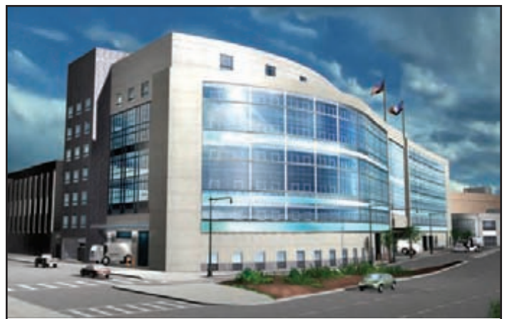
Future Manhattan District 4 Garage
