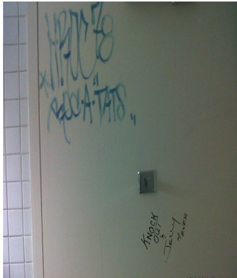
Service center bathroom door before CORE inspection
