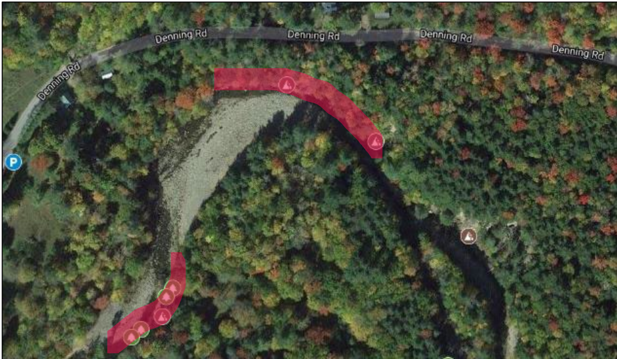
Figure 4. Aerial view of the Ladleton project site, with bank failure locations highlighted.
