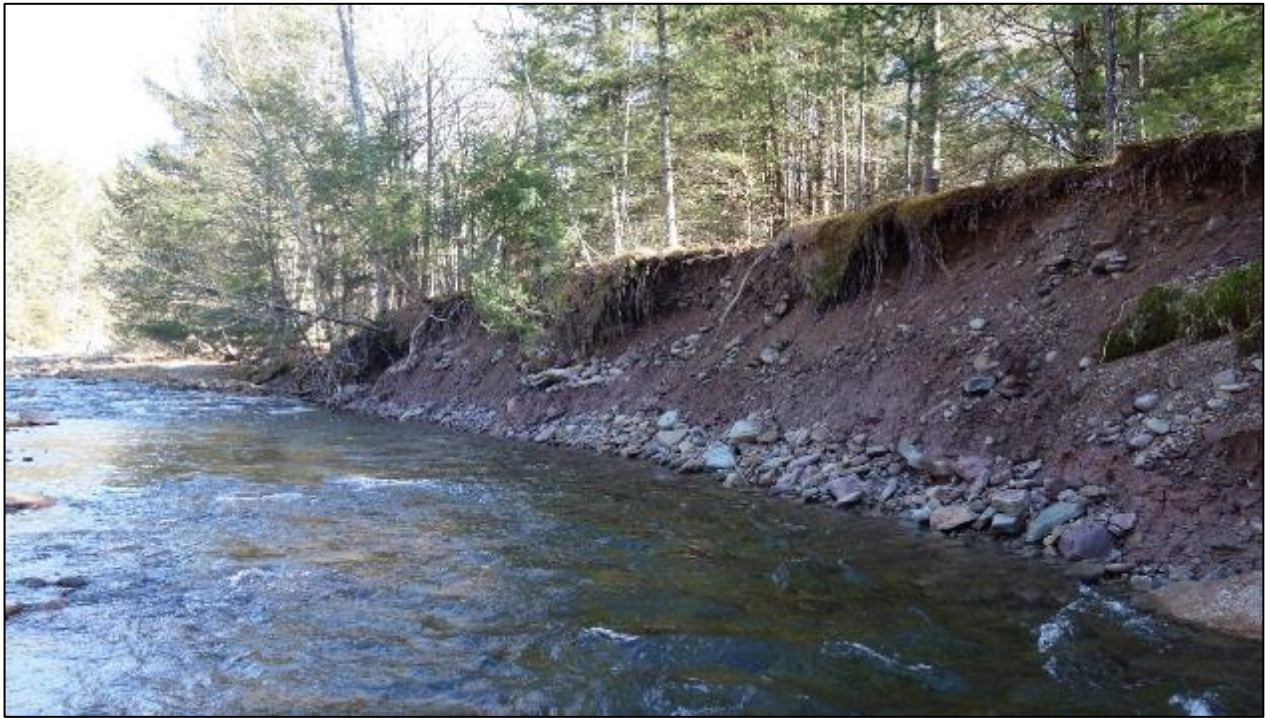
Figure 3. Secondary lower bank at the Ladleton project site.
