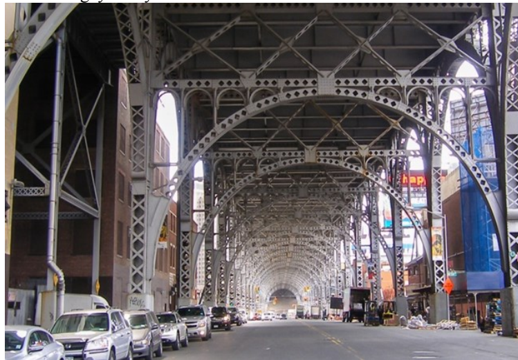
Protective coating of Riverside Drive Bridge over West 125th Street.
