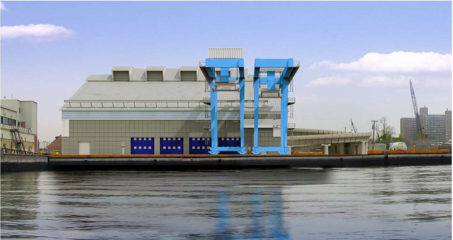
Southwest Brooklyn Marine Transfer Station
