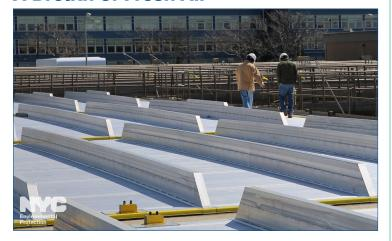
ast week, DEP announced that new odor control and air filtration systems have been installed at the Rockaway Wastewater Treatment Facility. As part of the approximately \$1 million project, 205 aluminum panels were installed over nearly 6,500 square feet of outdoor tanks where, as part of the treatment process, the wastewater is stirred up and can create odors. The air trapped under the covers will now be pulled from the tanks through
