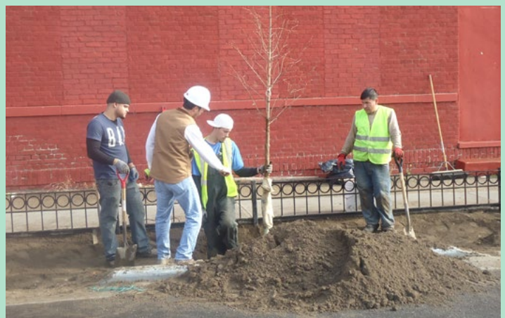
Right-of-way Bioswale tree planting, Junius St and Glenmore Ave., Brooklyn
