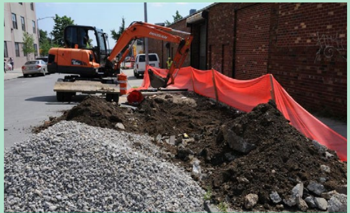
Right-of-way Bioswale construction, Junius St. and Liberty Ave., Brooklyn
