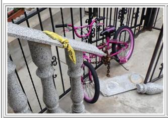
Contractors working in New York City should be advised that stone balustrade railings and fences can pose a serious hazard to the public, if they are not properly installed in accordance with the NYC Construction Codes.
