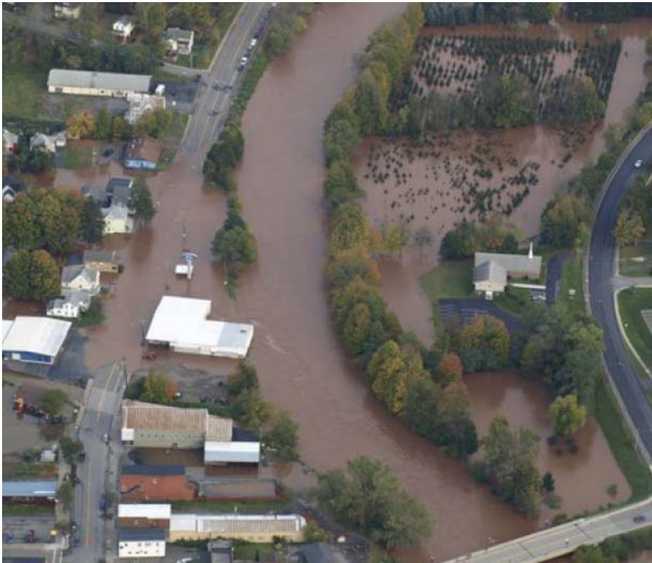
Figure 4: West Branch Delaware flooding at Walton LFA auto dealership site.
