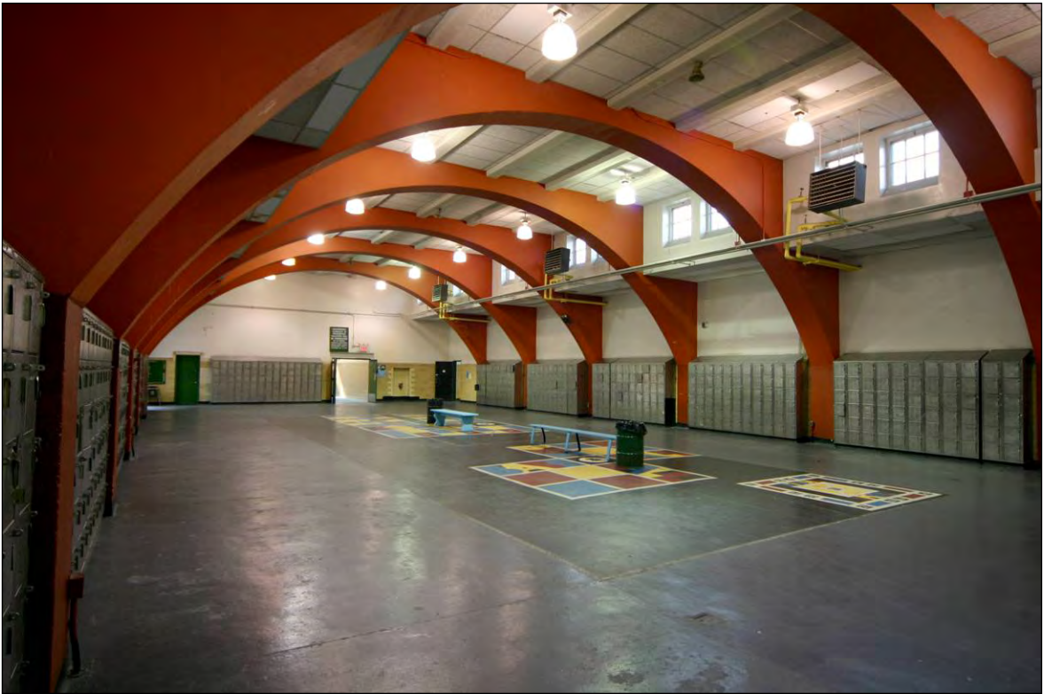
Crotona Play Center: Men's Locker Room Interior, South Wall (view southeast), Borough of the Bronx
