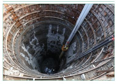
Construction continues on the outlet at Gilboa Dam where water released from the reservoir will be able to flow into Schoharie Creek below the dam. A gate shaft (above) is being bored at about the halfway point in the release tunnel. The gate shaft has to be blasted to a terminal depth of about 180 feet. Construction of the permanent release tunnel will allow the reservoir/dam to meet modern dam safety standards.
