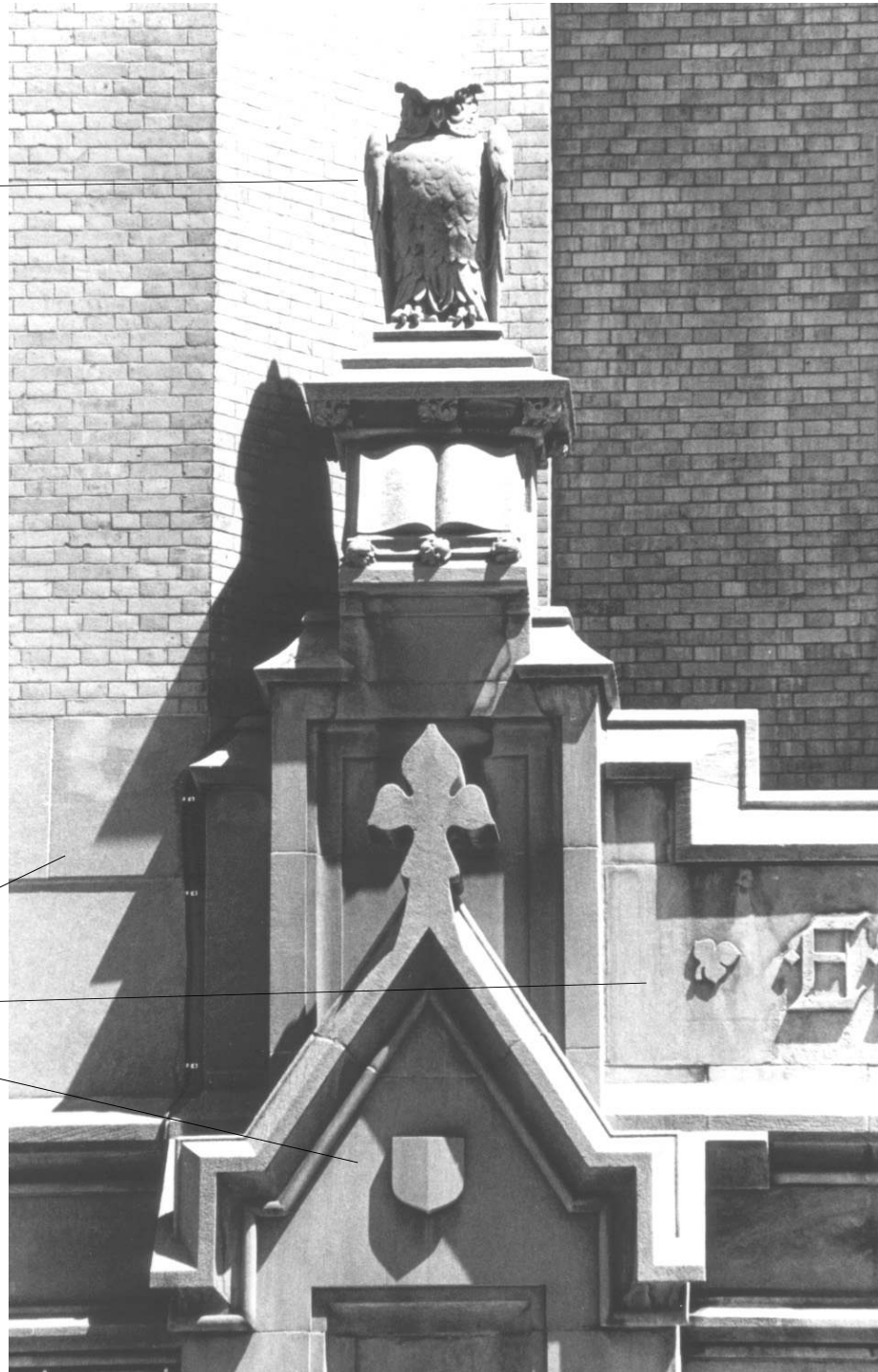
Erasmus Hall High School Tower A1 Detail of pier
