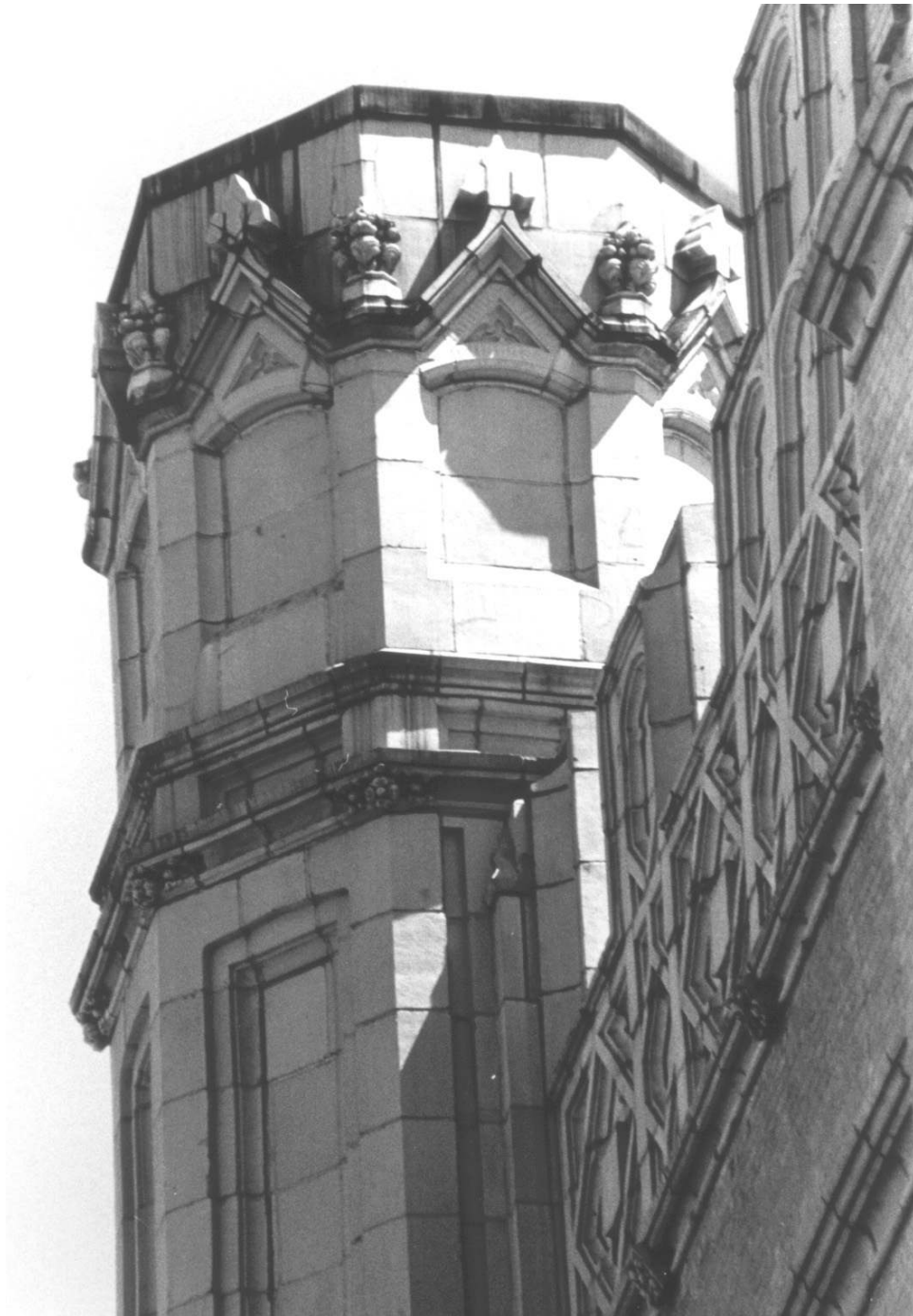
Erasmus Hall High School Tower A2 Terra-cotta detail of top of northern pier
