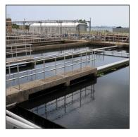
of pollutants and disease-causing pathogens from wastewater. The first step of the process is preliminary treatment, where a series of grates called bar screens remove solid objects—such as rags and pieces of wood that wash down storm sewers—from wastewater. Giant pumps then raise the wastewater to a series of settling tanks for primary treatment, another physical process in
