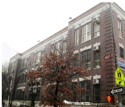
Main Entrance Facade facing Hicks Street
