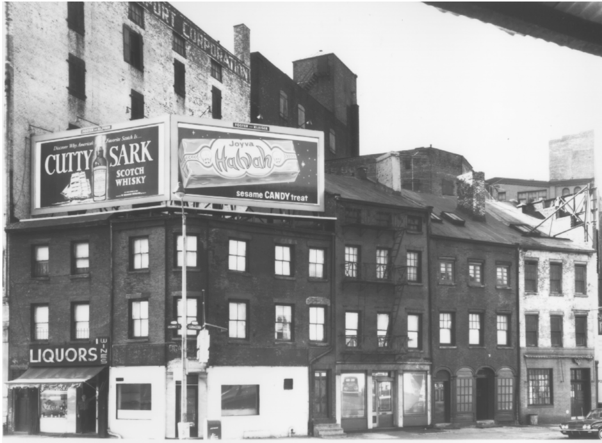
502, 504, 506, and 508 Canal Street, Manhattan Photo: John Barrington Bayley, 1965
