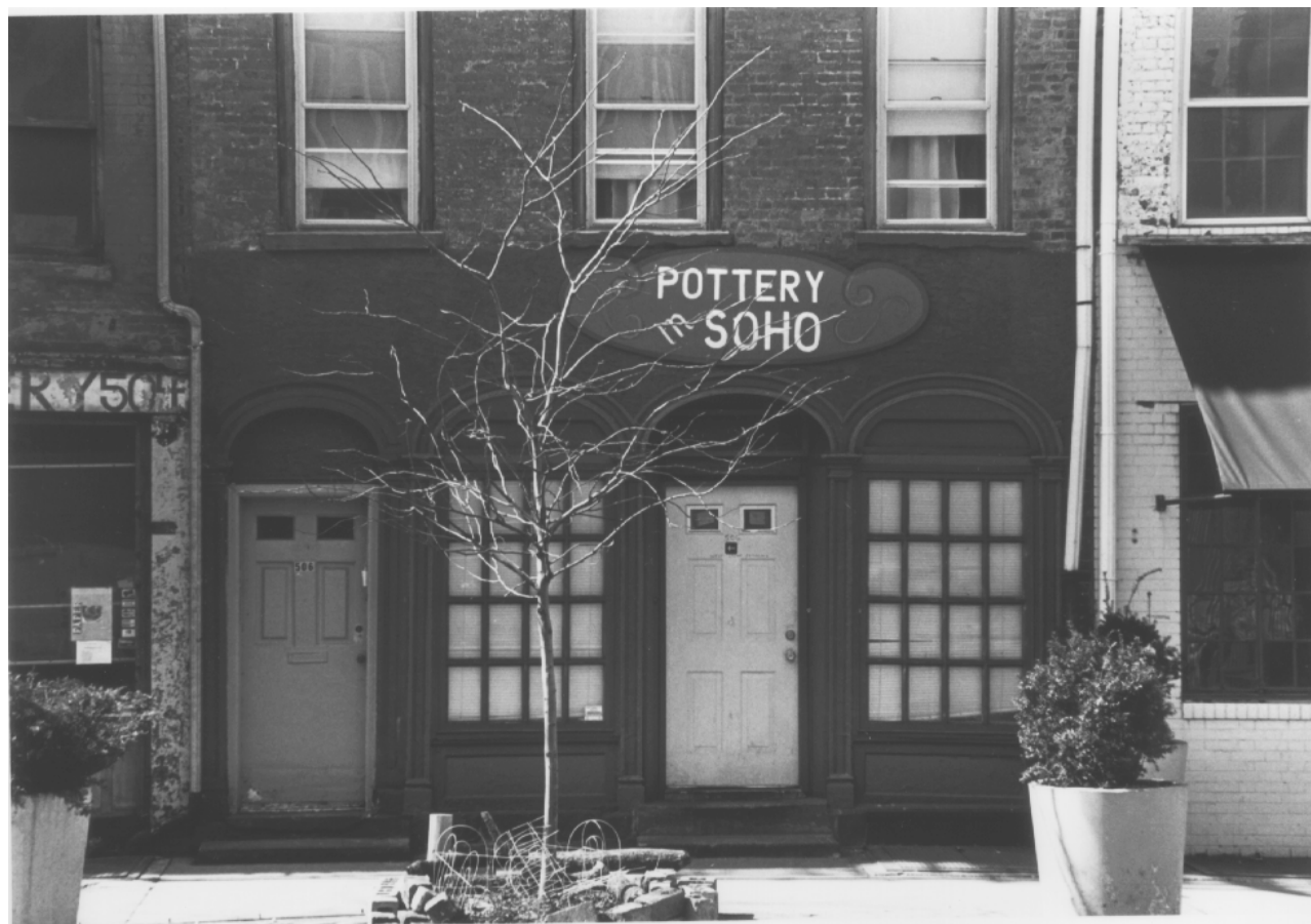
506 Canal Street House, Manhattan Storefront details Photo: Carl Forster, 1998
