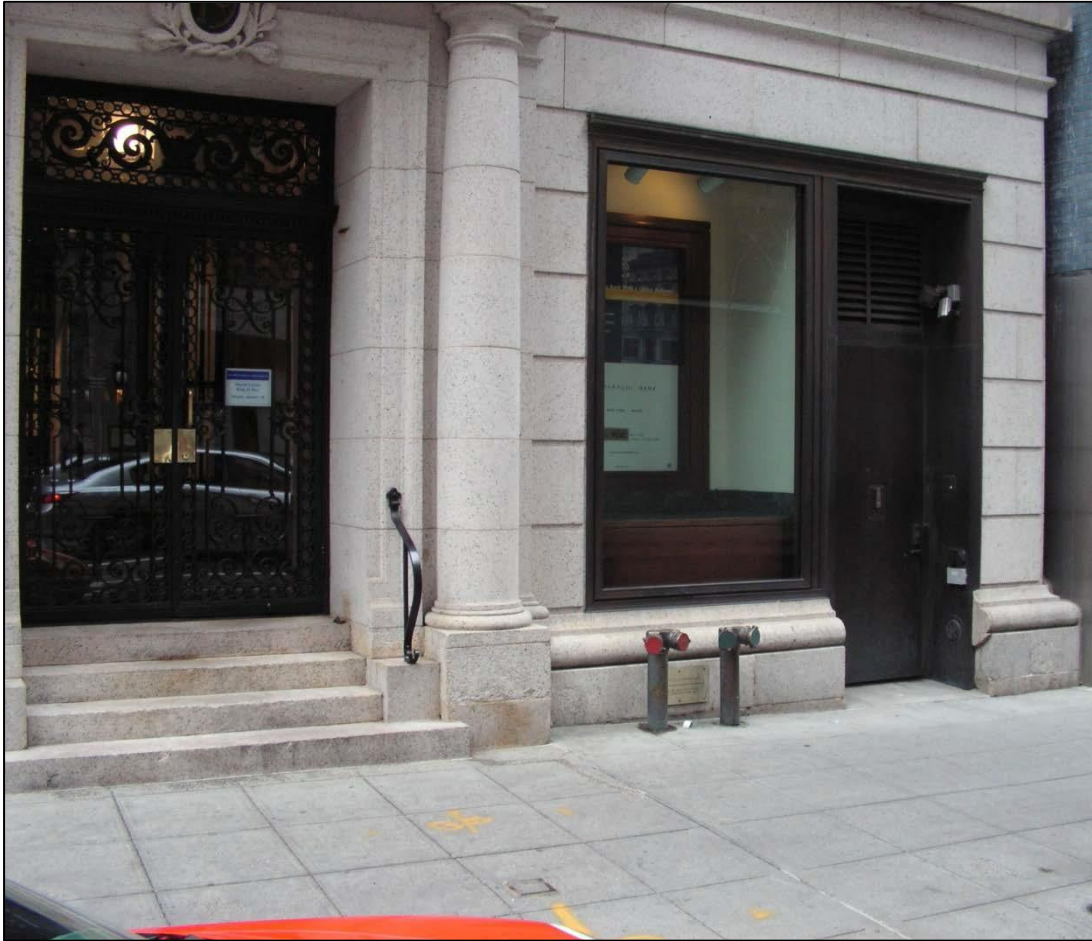
Minnie E. Young House 19 East 54 th Street Secondary entrance Photo: Theresa C. Noonan, 2016
