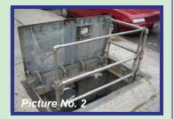
Newer installations might be equipped with "pop up" railings as seen in Photo No. 2. It is important to note that all four sides need to be guarded if the opening cannot be constantly guarded by an employee.
