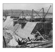
Then: Olive Bridge Dam during construction. The massive dam required a 30-foot trench filled with solid concrete and masonry in order to resist the constant pressure of 132 billion gallons of water attempting to push the dam into the valley. 12/8/1910
