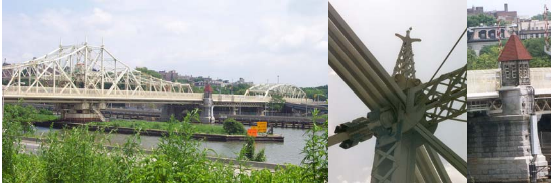
2004: East View of Macombs Dam Bridge Swing Span and Camelback Truss. (Credit: Peter Basich) Architectural Detail of the Bridge. (Credit: Michele N. Vulcan) Close-up of a Gate House. (Credit: Peter Basich)
