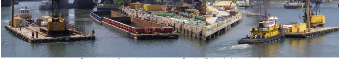
Construction Barge in June 2009. (Credit: Edgardo Montanez)
