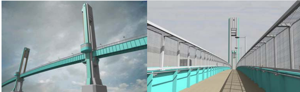
Proposed Fencing, Lighting, Access Platform and Handrail Along the Wards Island Bridge.
