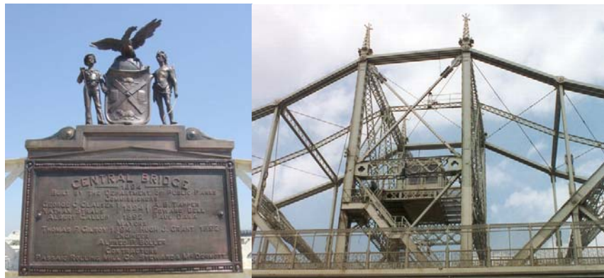
Close-up of the 1894 Dedication Plaque. (Credit: Hani Faouri) View of the Swing Span Control House. (Credit: Michele N. Vulcan)
