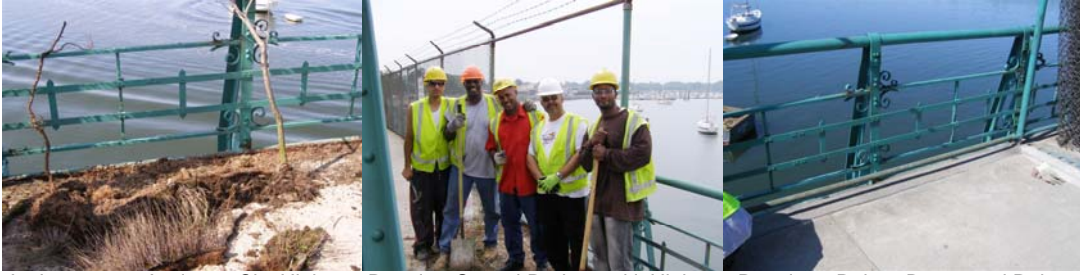
In June 2009, Assistant City Highway Repairer Seveul Redzeposki, Highway Repairers Robert Bynes and Ruben Sanchez, Supervisor Highway Repairer Dionisio Matos, and Assistant City Highway Repairer E'boni Brown Removed Vegetation From the Fascia Girder and Performed Chain Link Fence Repairs on the City Island Bridge. (Credit: Paul Schwartz)
