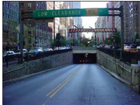
Park Avenue Tunnel in 2003. (Credit: NYSDOT)
