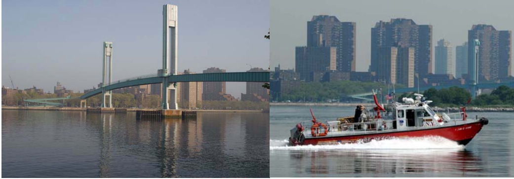
Wards Island Pedestrian Bridge After Completion of Painting in 2003. FDNY Rescue Boat Near the Bridge in 2008. (2008 Credit: Bernard Ente)
