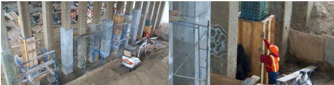
Pier 3 Column Repair in December 2008. (Credit: NYSDOT)
