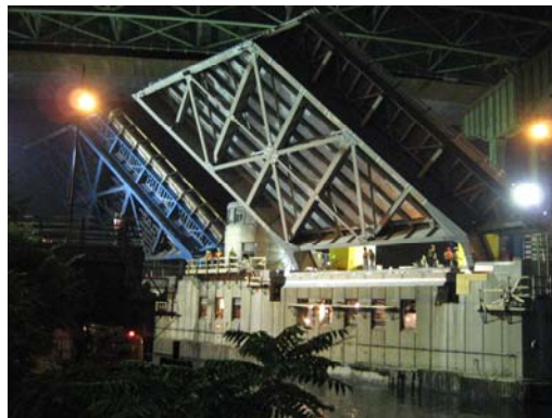
Open Hamilton Avenue Bridge in August 2007.
