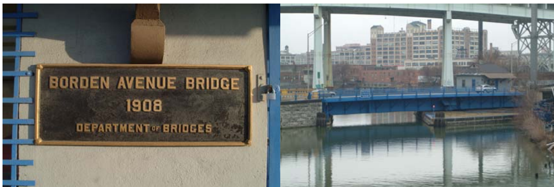
1908 Borden Avenue Bridge Plaque. Waterside View. (Credit: Bernard Ente)
