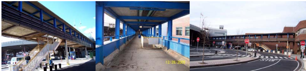
Pedestrian Breezeway - Over Commuter Drop-Off / Pick-Up Area.
