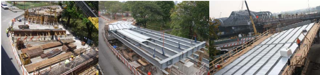
Temporary Loop Ramp in July and October 2008.
