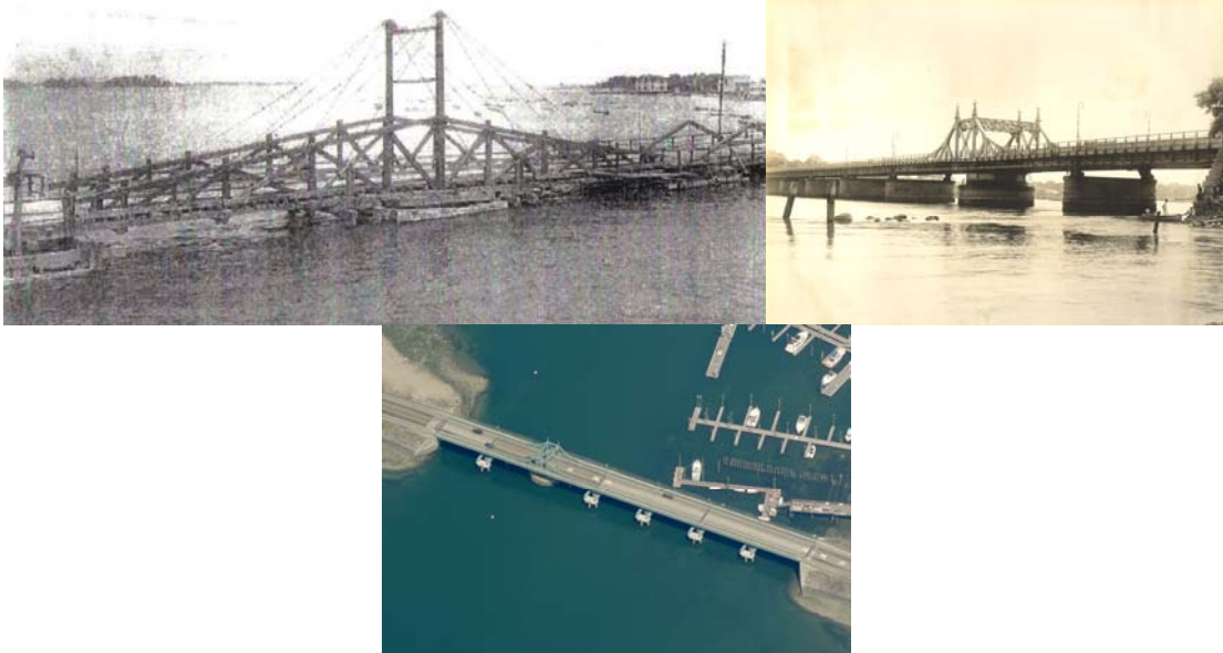
Original Bridge in 1873. Bridge in 1928. Aerial View of Current Bridge.
