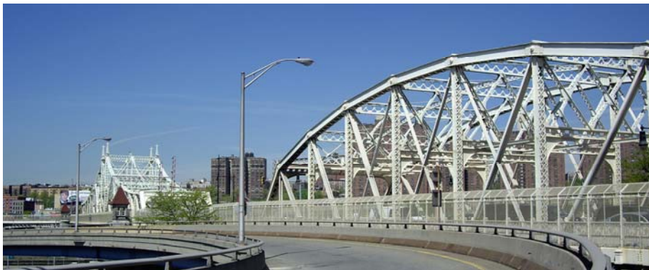
Macombs Dam Bridge in May 2007.
