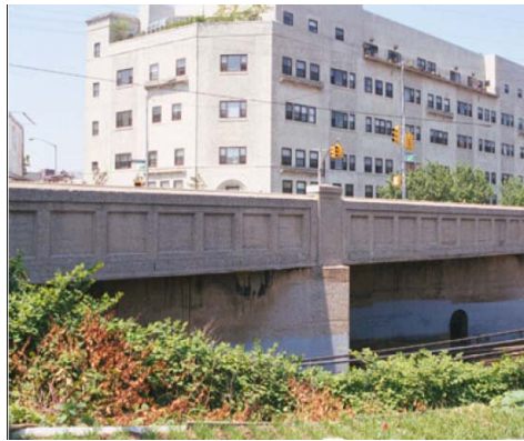
Woodside Avenue Bridge. (Credit: NYSDOT)
