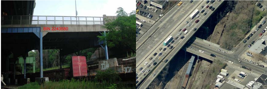
5 th Avenue Bridge in 2006. (Credit: NYSDOT) Aerial View in 2009.
