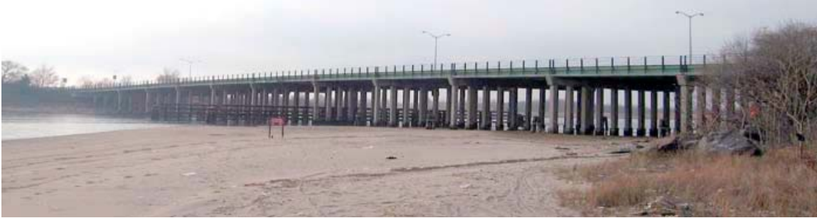
Paerdegat Basin Bridge.
