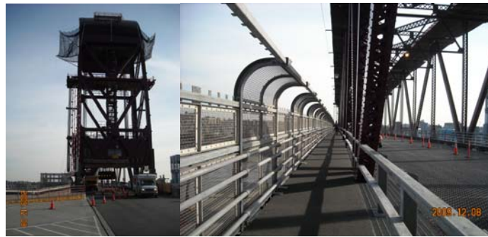
December 2008: Roosevelt Island Bridge West Tower West Elevation. Lift Span Sidewalk.
