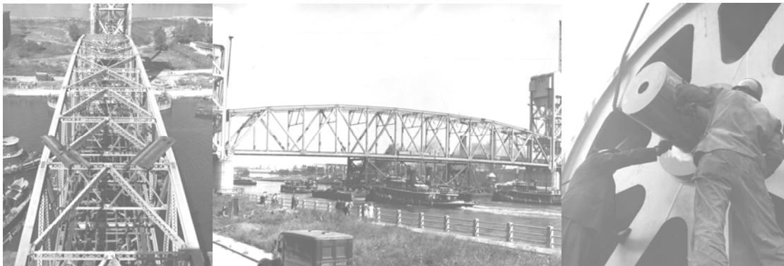
Roosevelt Island Bridge Under Construction in 1952.
