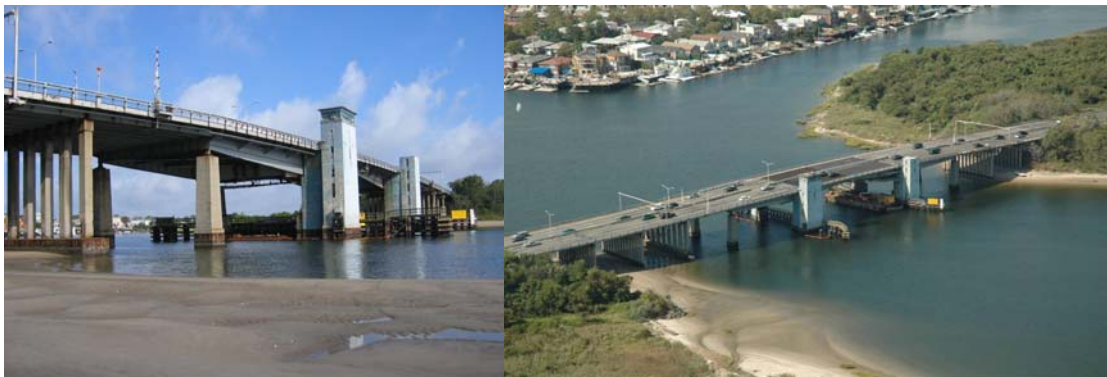
Belt Parkway Bridge Over Mill Basin. Aerial View.
