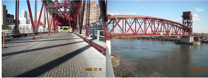
December 2008: Lift Span Open Grid Deck. Lift Span South Elevation.
