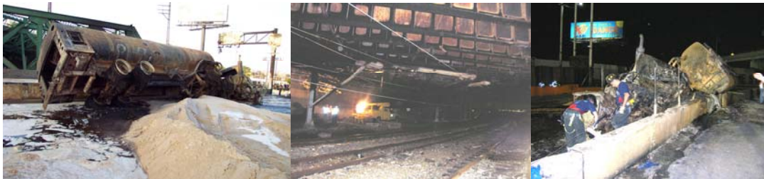
2005: The Tanker Truck. Repairs and Cleanup. (Credit: Bojidar Yanev)
