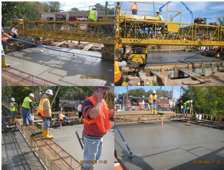
Annadale Road Bridge: Placing the Concrete Deck in October 2008.
