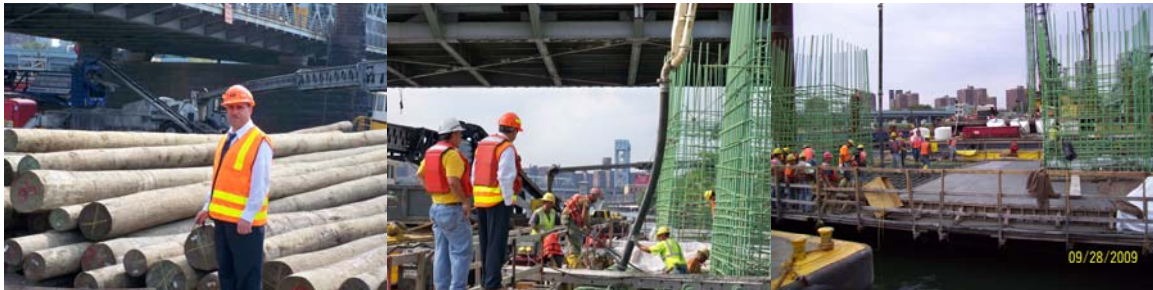
September 2009: Administrative Engineer Hani Faouri at Pier 7. Pier 7 Box Concrete Infill.
