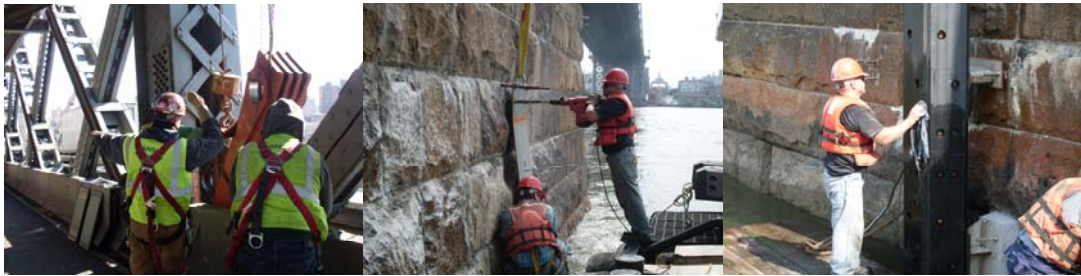
Contract #8 in 2009: Looking Southeast at the Installation of the Triangular Jacking Frame for the Intermediate Tower Bearing Replacement in January 2009. Main Tower Pier Fender System Installation in July 2009.
