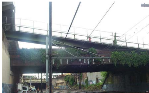
Bryant Avenue Bridge in 2002. (Credit: NYSDOT)
