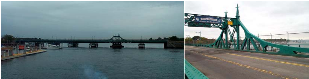
City Island Road Bridge. Vertical Clearance Posting. (Credit: NYSDOT)
