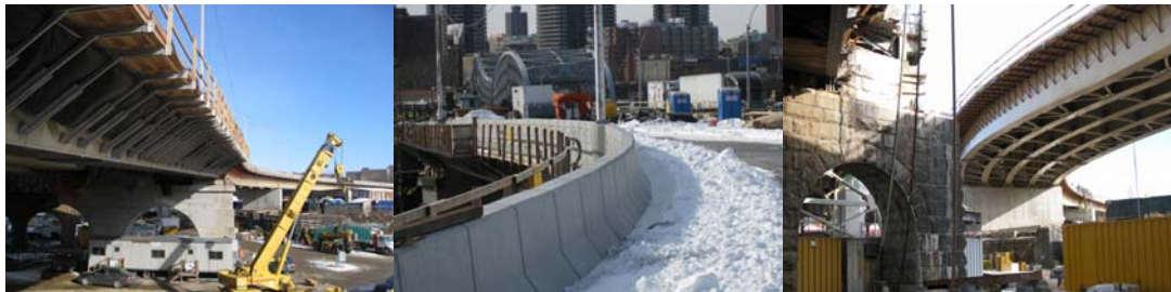
Construction Site in December 2009. (Credit: Brian Gill)
