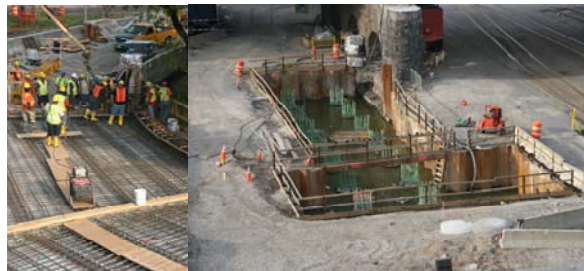
Temporary Loop Ramp in October 2008. Pier 9 Drilled Shaft Footing in November 2008.
