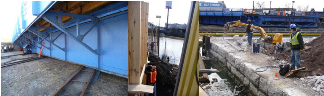
Borden Avenue Bridge in February and March 2009. (Credit: Tamara Berlyavsky)
