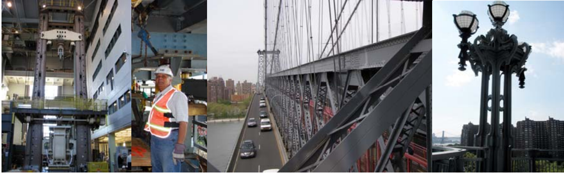
Contract #8 in 2009: Testing the Intermediate Tower Bearings at Lehigh University in January 2009. Assistant Engineer-in-Charge Anil Rudra on the Bridge in July 2009. Resurfaced South Outer Roadway. (Roadway Credit: Bojidar Yanev). Looking South at the Manhattan Main Tower Electrolier in December 2009.
