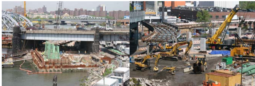
May 2009: Willis Avenue Bridge Construction Site. FDR Drive Ramp Demolition.
