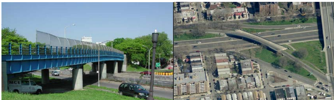
East 8 th Street Bridge in 2002. (Credit: NYSDOT) Aerial View in 2009.
