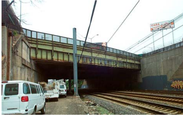
Bruckner Expressway Bridge NB in 2002. (Credit: NYSDOT)
