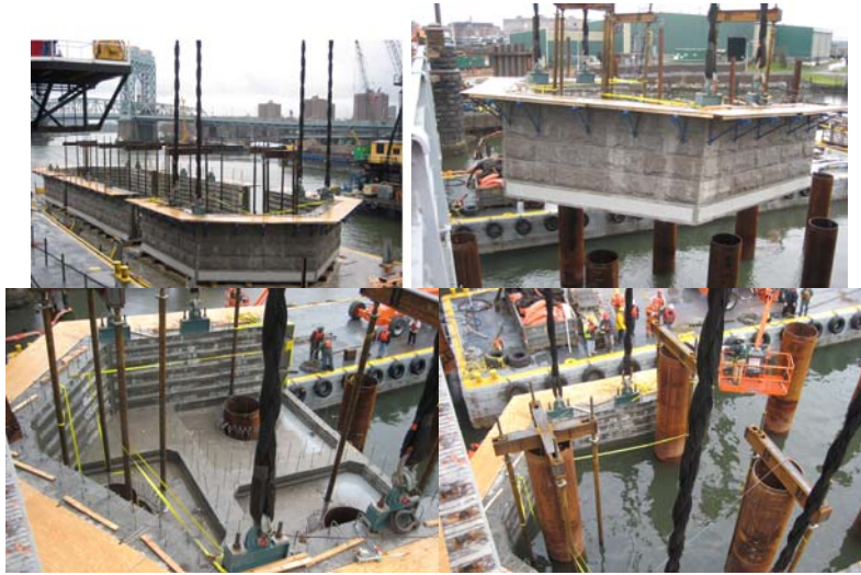
The First River Pier in November 2008.
