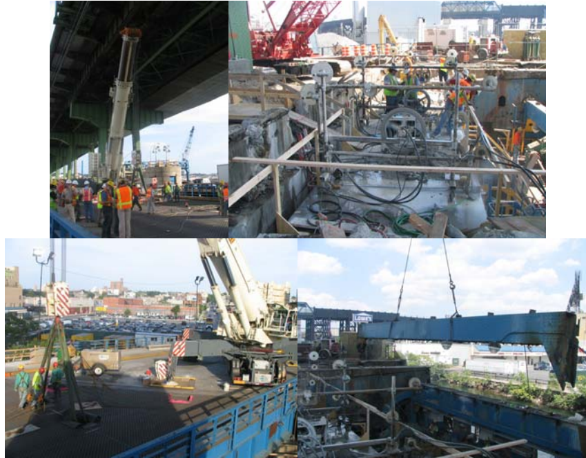
Removing the East Span in July 2007.
