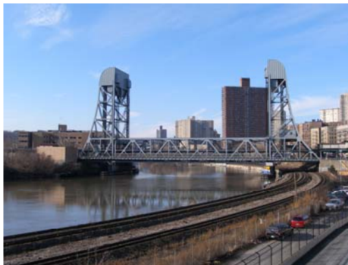
Broadway Bridge in December 2008. (Credit: Sergey Parayev)
