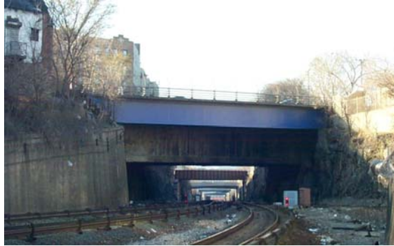
Grand Concourse Bridge over Metro North in 2002. (Credit: NYSDOT)
