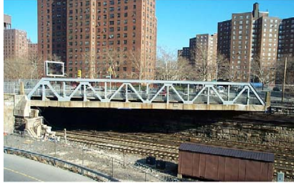
Concourse Village Avenue Bridge. (Credit: NYSDOT)
