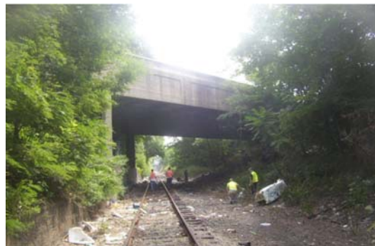
50 th Street Bridge in 2003. (Credit: NYSDOT)
