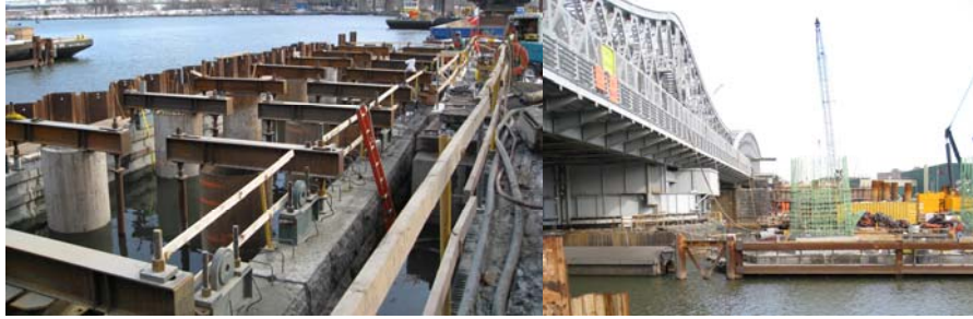
Construction Site in December 2009. (Credit: Brian Gill)
