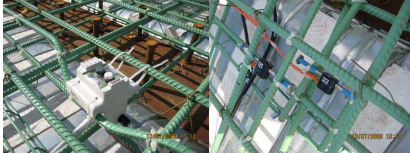
The Embedded Corrosion Instrument Sensor is a Non-Destructive Evaluation Instrument. The Variable Wire Strain Sensor Gauges Strain.
