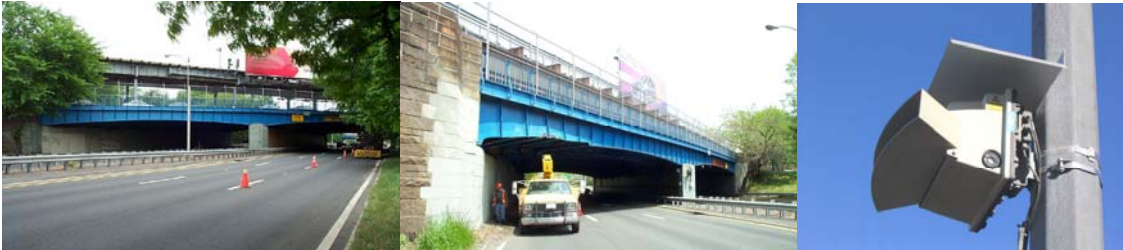
Westchester Avenue Bridge in 2001 and 2006. (Credit: NYSDOT) Overheight Sensor Unit on the Hutchinson River Parkway. (Credit: Roly Parroco)
