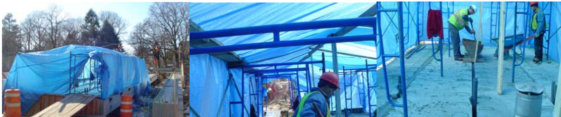
Grouting of the West 252 nd Street Bridge Box Beams in February 2007.
