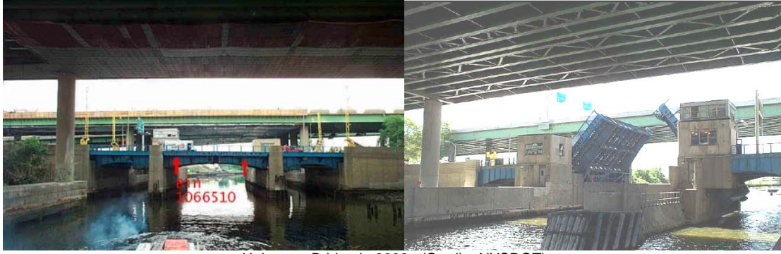
Unionport Bridge in 2002. (Credit: NYSDOT)
