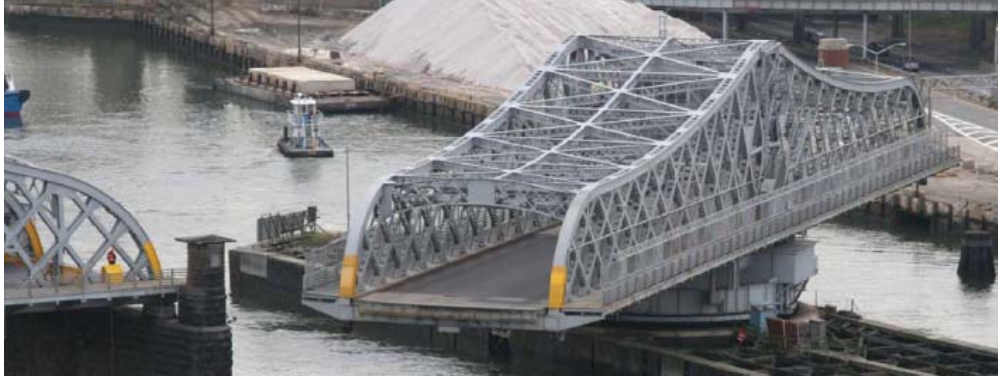
Open Willis Avenue Bridge.
