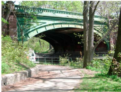
Hill Drive Bridge in 2001. (Credit: NYSDOT)
