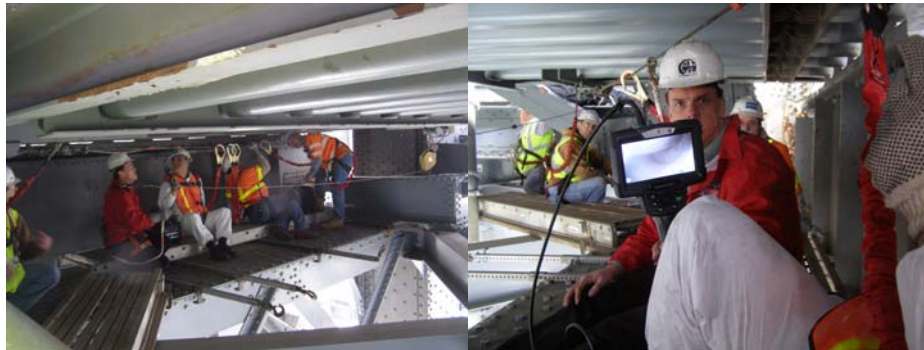
Director of Bridge Management Kevin McAnulty (in Red Jacket) Utilizing a BoreScope to Inspect the Joints of the Williamsburg Bridge in April 2009.
