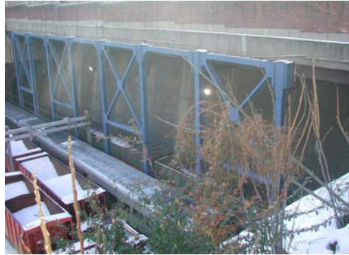
West 31 st Street Bridge in 2004. (Credit: NYSDOT)
