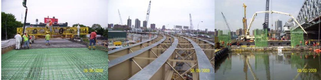
Willis Avenue Bridge August 2009: Placement of Deck Concrete on New Ramp to Bruckner Boulevard. Curved Girders on New Ramp. Placing Concrete in Pier 7 Box.
