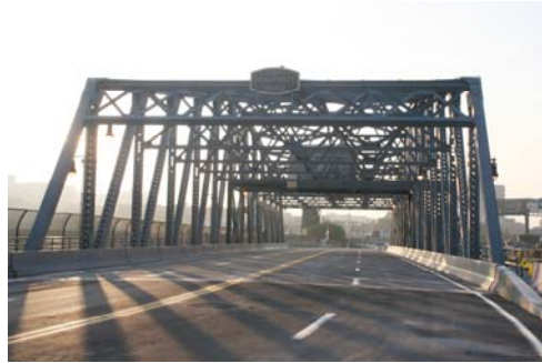
2007: New Bridge Ready for Traffic.
