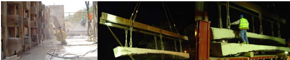
2006: Cutting and Removing the Existing West 252 nd Street Bridge Sections Over the Parkway.
