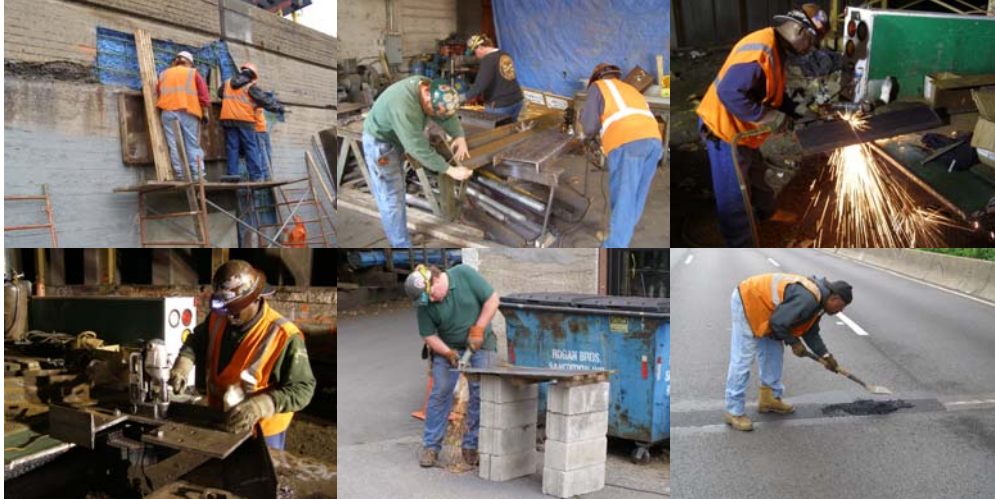
Repairs at the Henry Hudson Parkway Viaduct in May and June 2009.
