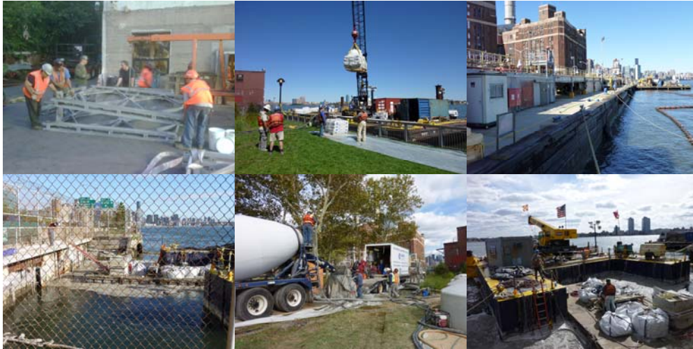
Emergency Repairs on the FDR Drive in August and September 2009.
