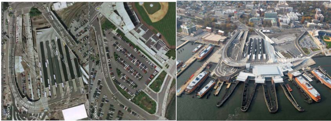
Aerial Views of the Staten Island Ferry Terminal Ramps.
