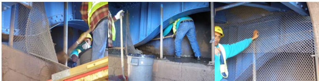
Highway Repairer Ruben Sanchez Cleaning the 174 th Street Bridge Seat. (Credit: Louis Garzia)
