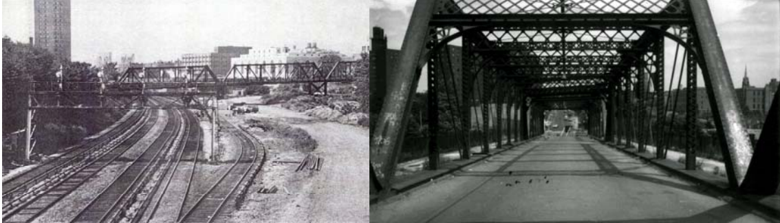
Original 153 rd Street Bridge. Bridge in Early 1980's.
