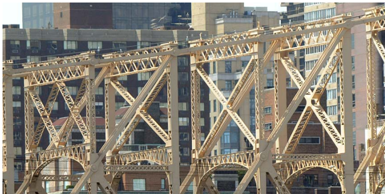
Bridge Detail in 2008. (Credit: Bernard Ente)
