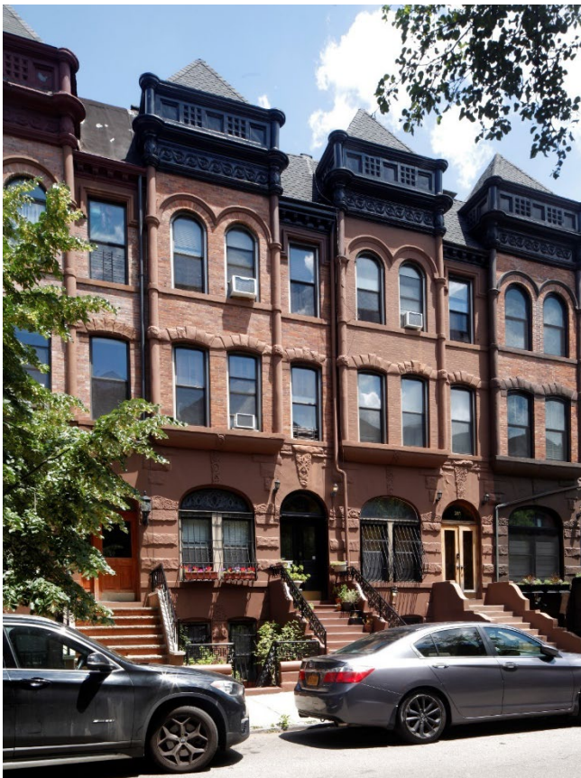
Figure 11 Houses in the row from 225 through 265 West 136th Street Jessica Baldwin, LPC, 2021
