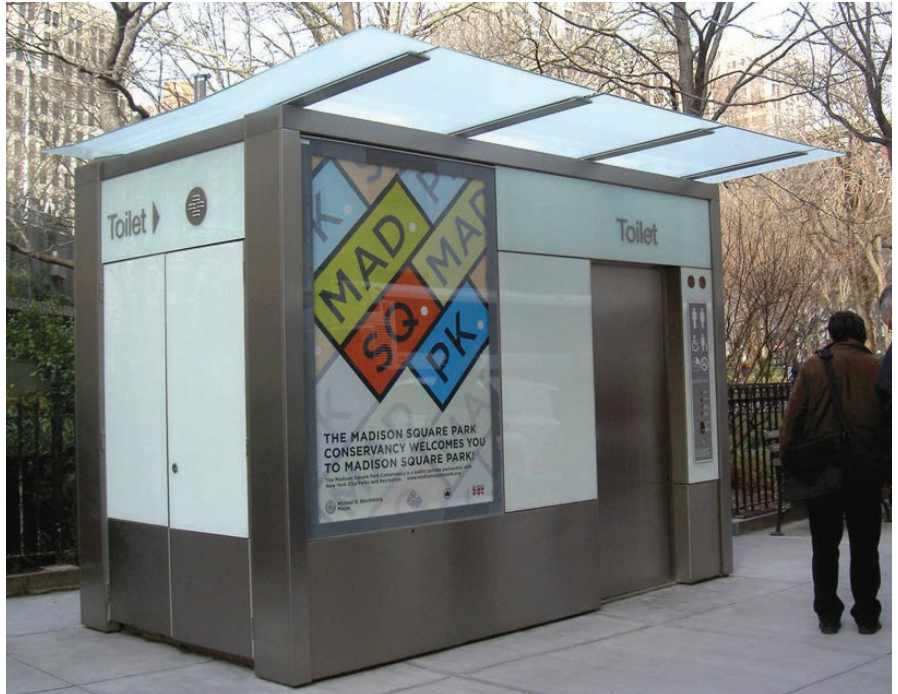
Madison Avenue at 23rd Street, Manhattan (Credit: Cemusa, Inc.)
