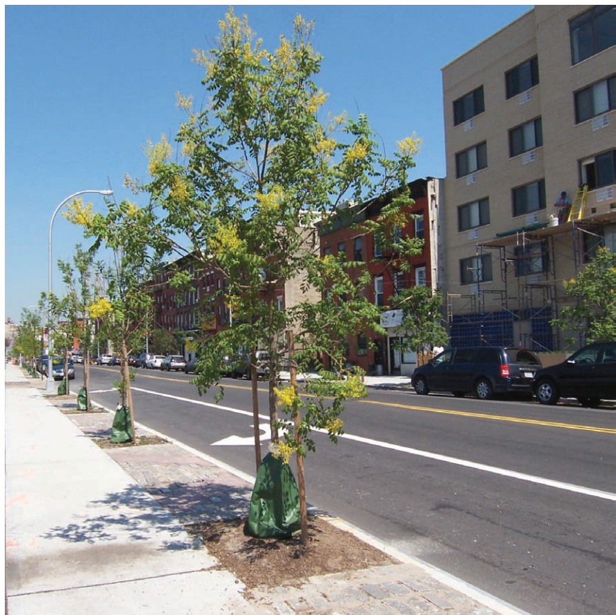
Connected tree beds with permeable-paver-covered trench: Columbia Street, Brooklyn (Credit: DPR)
