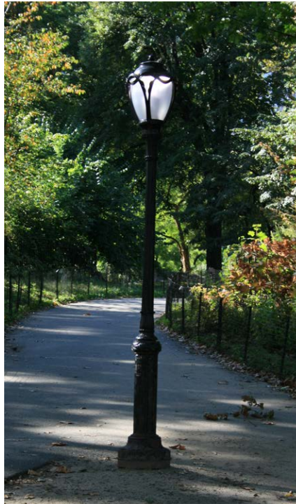
Type B luminaire and pole with LED lamp
