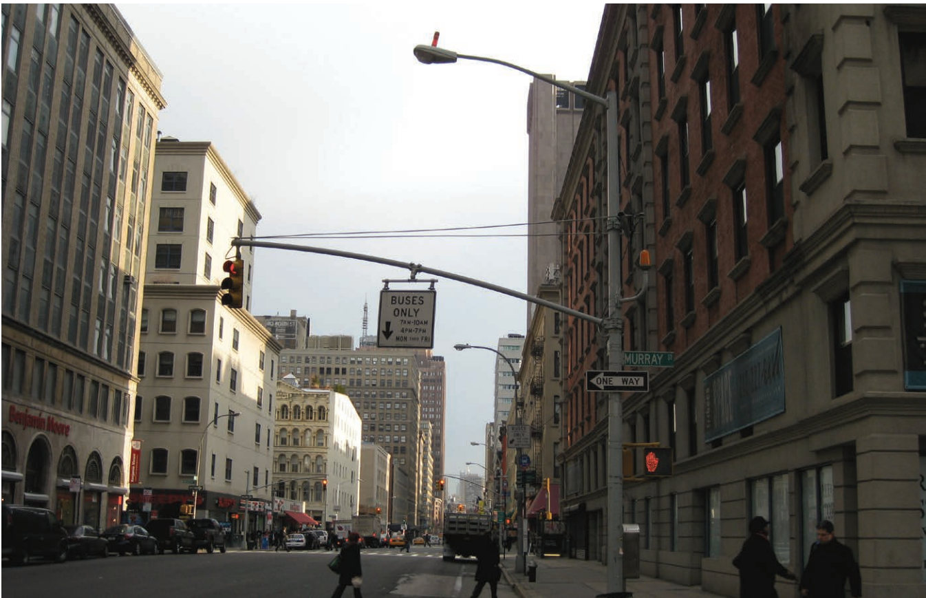
Type M-2A signal pole with HPS Cobra Head luminaire: Murray Street, Manhattan
