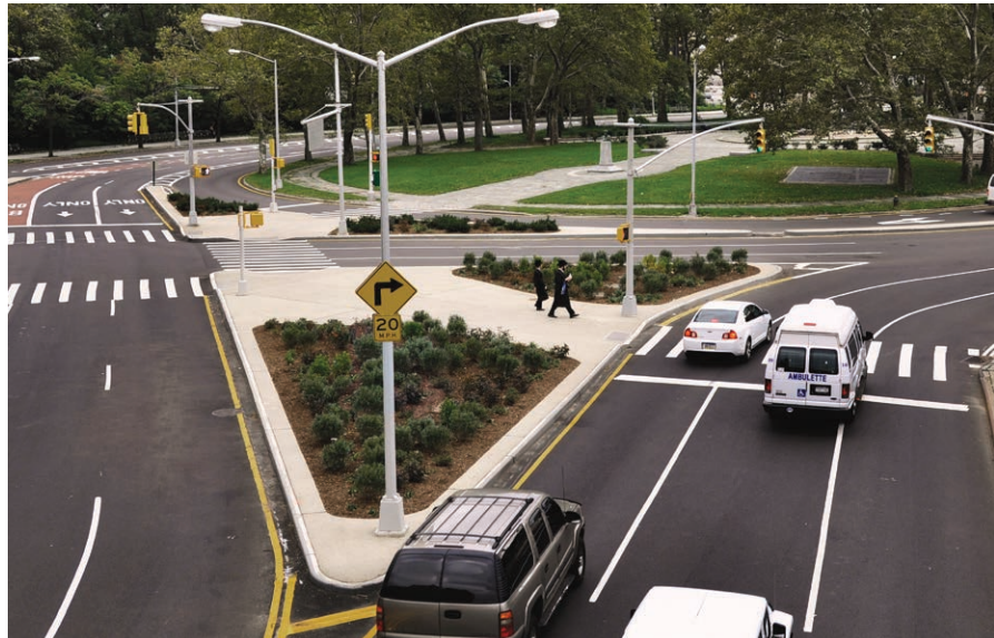
Planted triangle. Clear paths are provided for pedestrian circulation: Grand Army Plaza, Brooklyn
