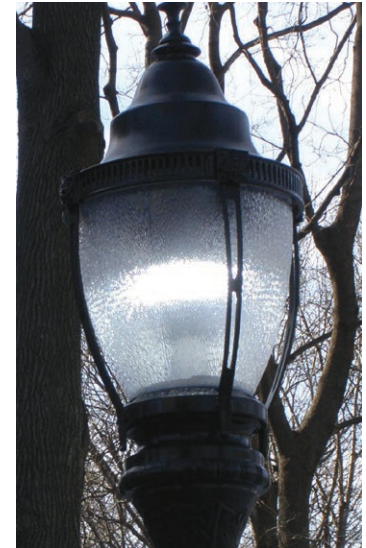
Type B luminaire and pole with LED lamp
