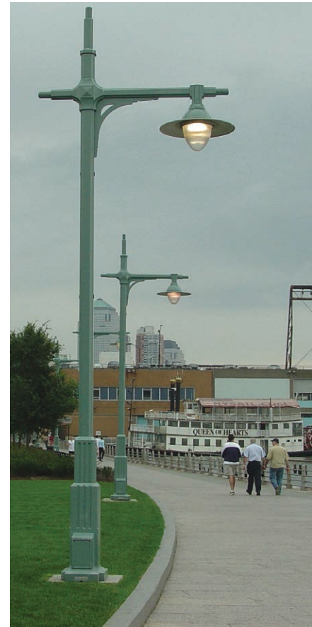
TBTA pole with Historic Shielded Teardrop luminaire: Hudson River Park, Manhattan
