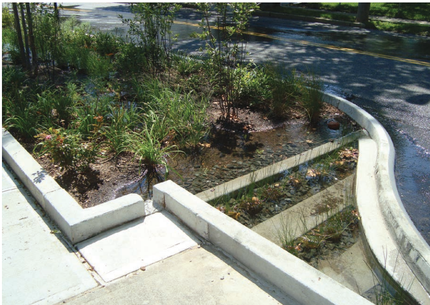
Water can be collected in a forebay, such as the triangular area shown on the right. This allows sediment and debris to settle before the water continues to the planting area: Westbourne Avenue at Bay 25th Street, Queens (Credit: DPR)
