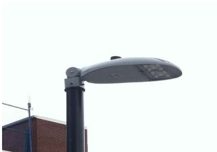
Standard LED Luminaire on Flushing Meadows Pole: Putnam Plaza, Brooklyn
