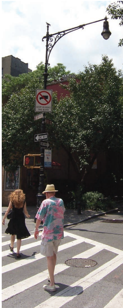
Historic Type M luminaire and pole: West 11th Street, Manhattan
