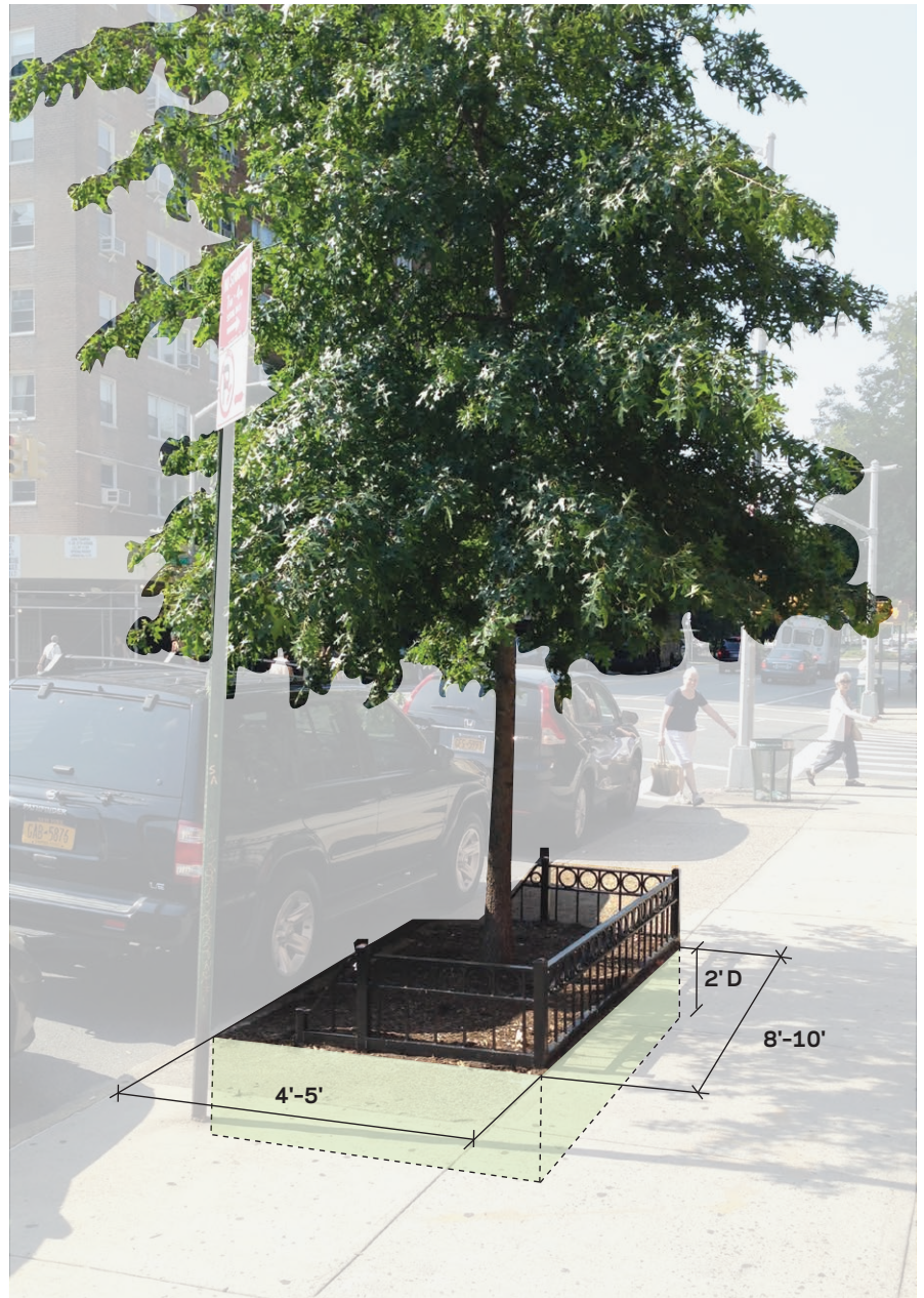
Tree bed with standard tree-bed guard. While tree beds may vary in size, larger dimensions allow for more growth: Vanderbilt Avenue, Brooklyn
