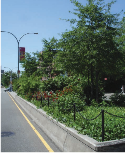
Raising medians to over 12 inches helps accommodate tree roots: West Houston Street, Manhattan (Credit: DPR)
