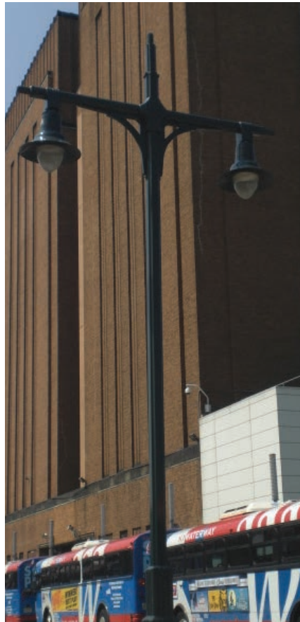
TBTA pole with Historic Shielded Teardrop luminaires: 40th Street, Manhattan
