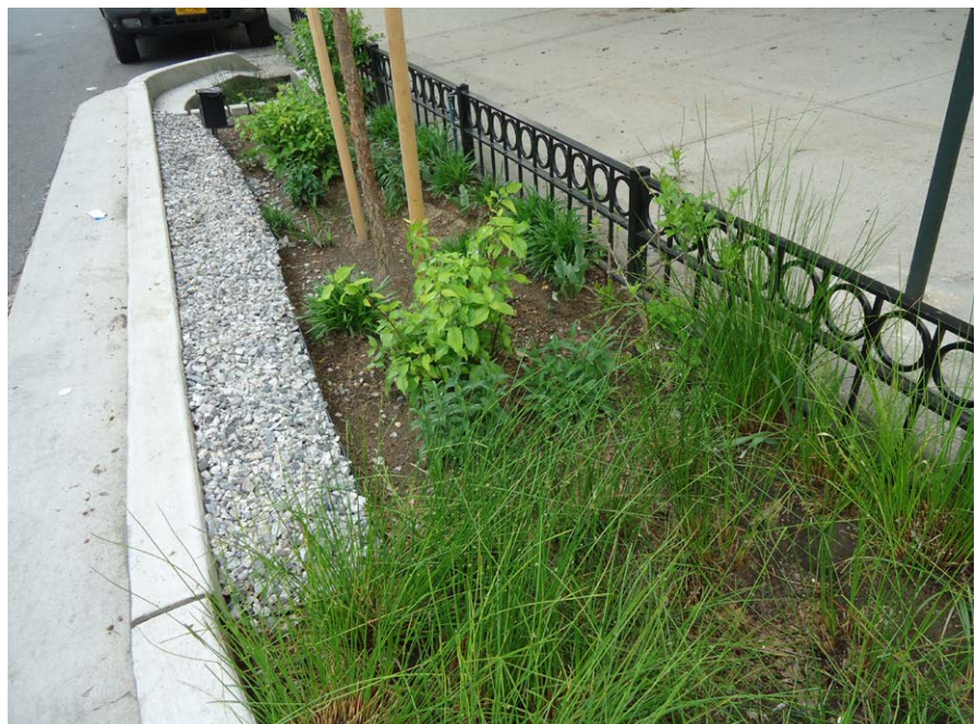
DEP ROW Stormwater Greenstreet constructed in the roadway, modifying the street geometry: Powell Street and Belmont Avenue, Brooklyn (Credit: DEP)
