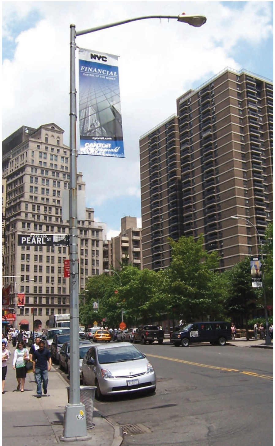
Octagonal pole with HPS Cobra Head luminaire: Pearl Street, Manhattan
