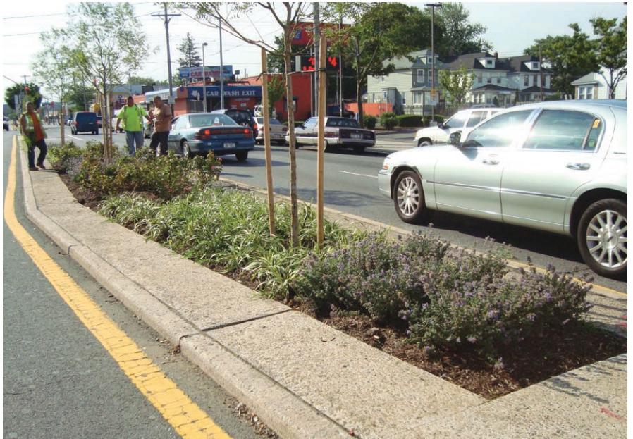
Curb-height median with plantings set back from the curb to allow for easier maintenance: Merrick Boulevard, Queens (Credit: DPR)
