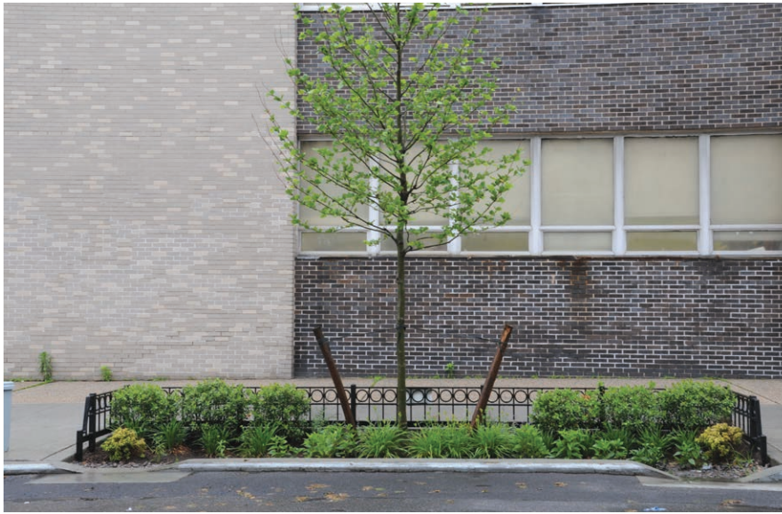
Typical DEP ROW Bioswale with tree: 62nd Drive and Junction Boulevard, Queens (Credit: DEP)
