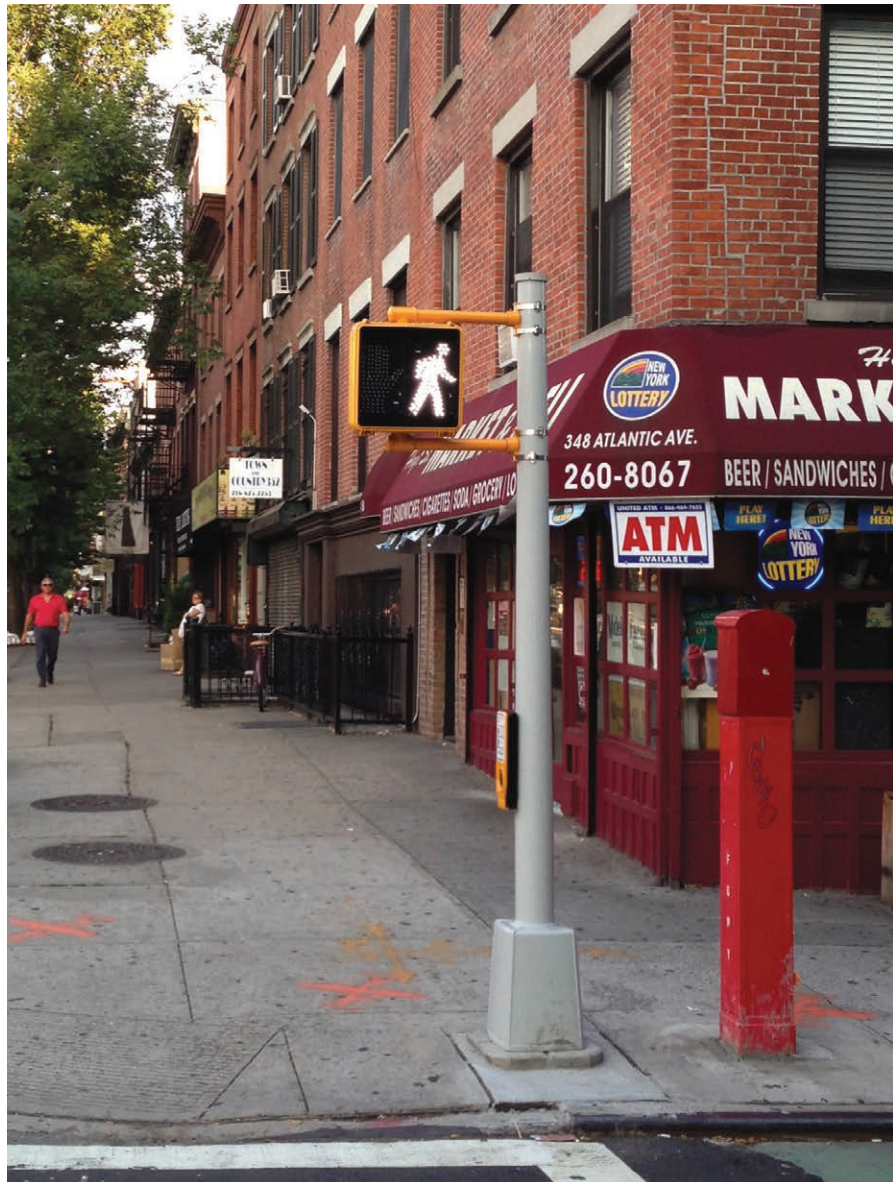
Type S-1A signal pole with a pedestrian signal: Hoyt Street, Brooklyn
