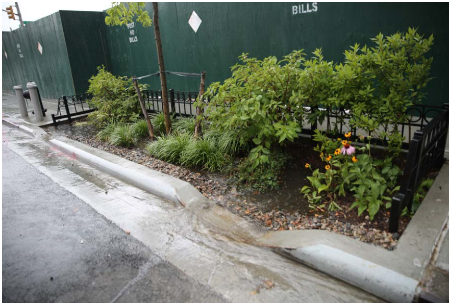
Stormwater entering DEP ROW Bioswale through inlet and overflow exiting from outlet: Dean Street and 4th Avenue, Brooklyn (Credit: DEP)
