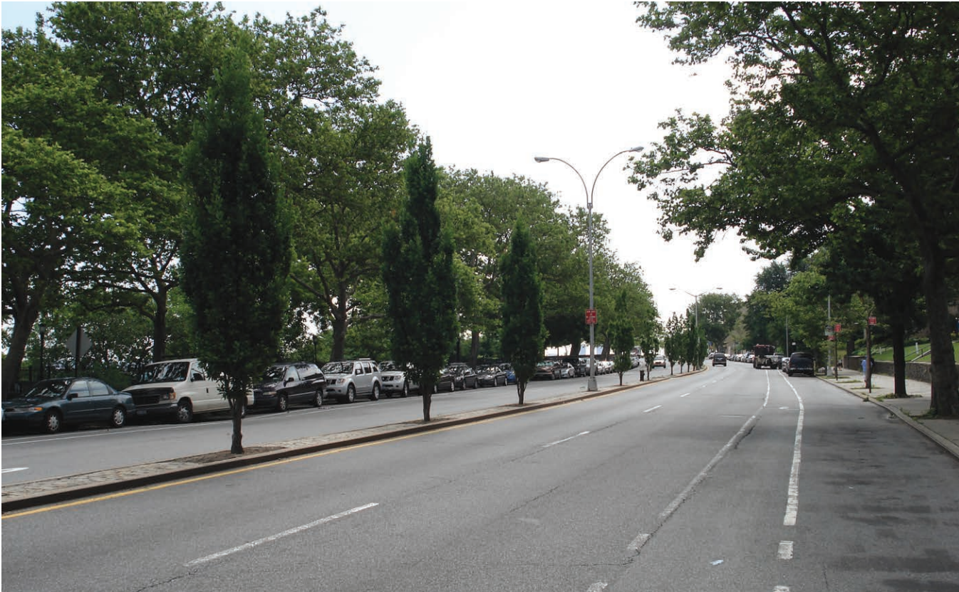
Curb-height median with tree beds. Select narrow species where there is limited space for canopies: Richmond Terrace and Nicholas Street, Staten Island (Credit: DPR)
