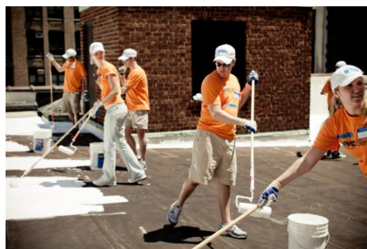
On average, for every 2,500 square feet of roof that is coated, the city's carbon footprint can be reduced by 1 ton of CO 2 e.
