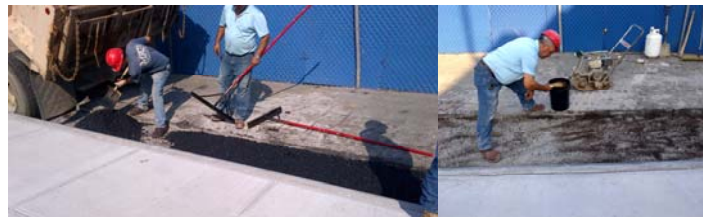
May 2012: Application of Binder Course and Tack Coat.
