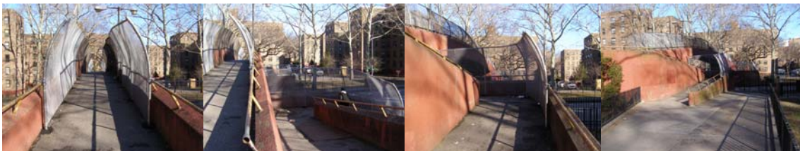
Additional Fencing on the Pedestrian Bridge.
