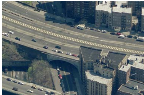
Grand Concourse Bridge over East 174 th Street in 2007.
