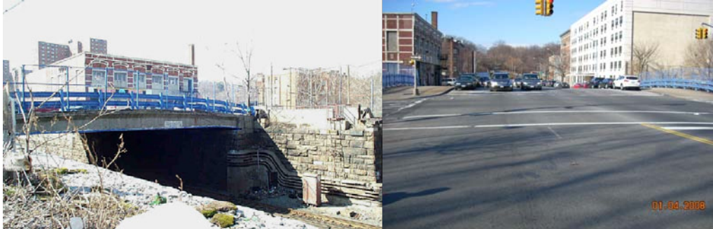
Claremont Parkway Bridge. (Credit: NYSDOT) Looking Northwest in 2008.
