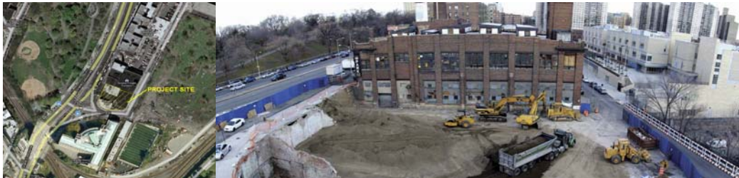
Grand Concourse Project Site. During Demolition in Winter 2012.
