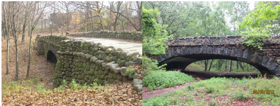
Highland Park Bridge.
