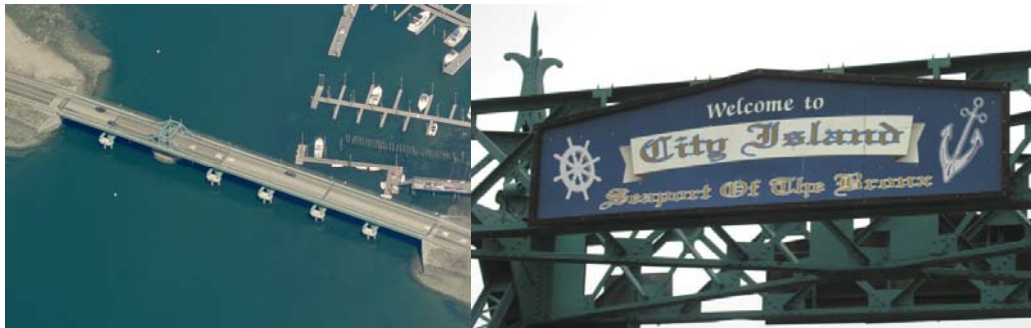
Aerial View of Current Bridge. Welcome Sign.
