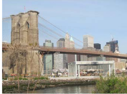
December 2012: Brooklyn Main Span in Finish Coat.
