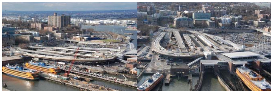
December 2012: Project Site.
