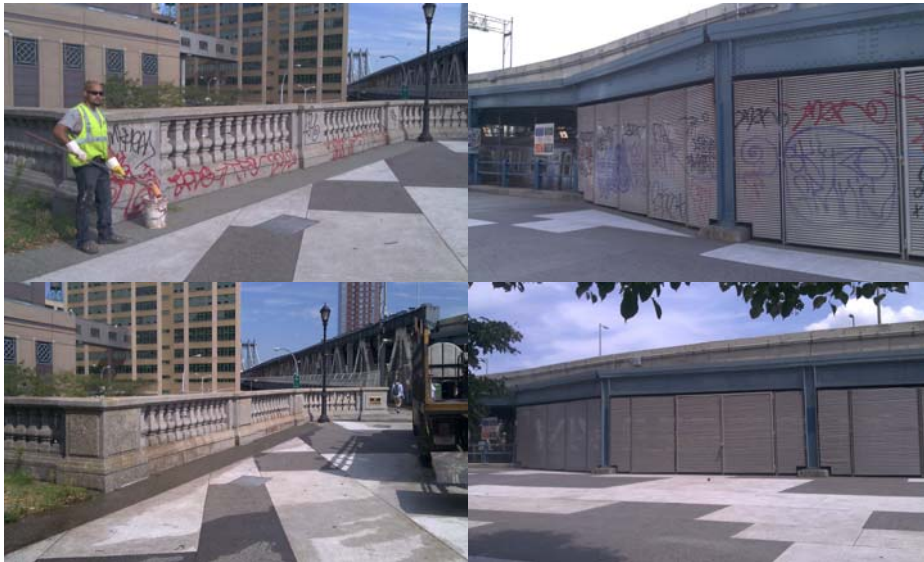
Bridge Painter Herbert Rodriguez and Before and After Graffiti Removal on the Manhattan Bridge in August 2012. (Credit: Robert Avellino)
