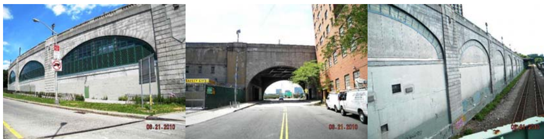
Riverside Drive Bridge in 2010. (Credit: NYSDOT)
