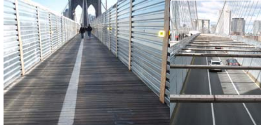
Bicycle/Pedestrian Path with Protective Shielding in November 2010. Roadway Shielding in October 2010.
