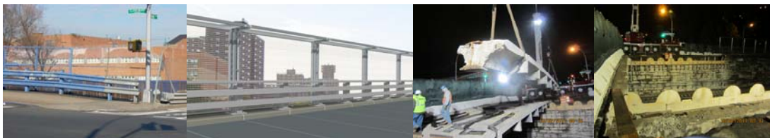
Existing North Side Guardrail and Fence. Proposed Guardrail and Fence. Stage 1 in October 2011: Removal of the Existing Bridge Girders.
