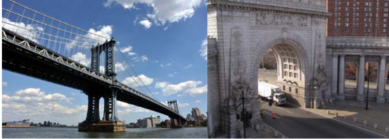
Manhattan Bridge in July 2009. (Credit: Bernard Ente) Arch and Part of the Colonnades in March 2011. (Credit: Bojidar Yanev)
