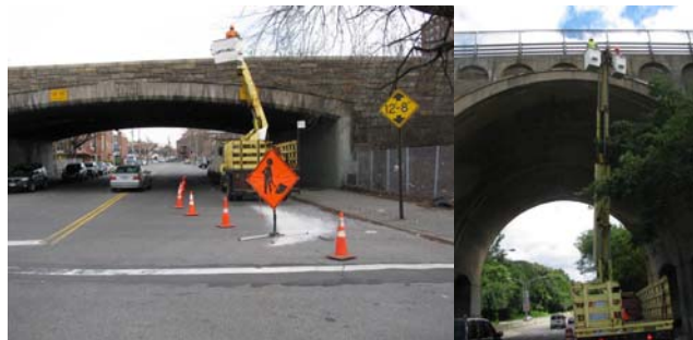
Inspecting the Belt Parkway Bridge over 26 th Avenue in December 2012. (Credit: Artemio Angeles) Inspecting the Nereid Avenue Bridge over Bronx River Parkway in June 2012, Using a 60 Foot Boom With Outriggers. (Credit: Bojidar Yanev)
