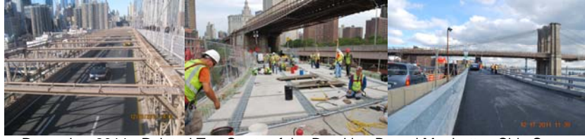
December 2011: Painted Top Struts of the Brooklyn-Bound Manhattan Side Span. Summer 2011: Manhattan Approach - Ramp C Deck Replacement. December 2011: Ramp C.
