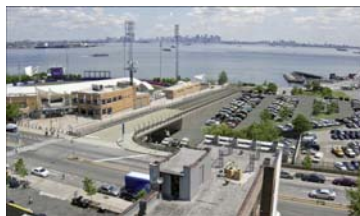
June 2012: New North Ramp.
