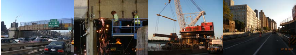
Removal of the Old Bridge in July 2011.
