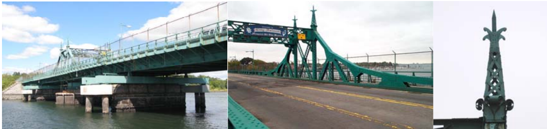
City Island Road Bridge in 2010. (Credit: Bojidar Yanev) Vertical Clearance Posting. (Credit: NYSDOT) 9 Foot Tall Ornamental Finial.
