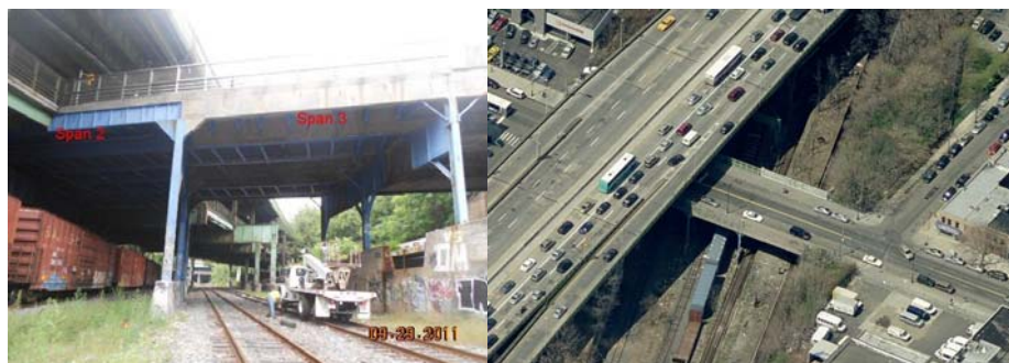
5 th Avenue Bridge in 2011. (Credit: NYSDOT) Aerial View in 2009.
