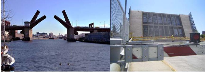
Pulaski Bridge Opening in February 2010. (Credit: Bernard Ente) Third Street Bridge Opening in June 2012. (Credit: Nikita Gupta)
