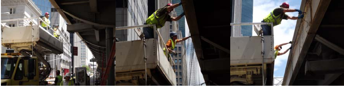
Installing Pigeon Netting at Old Slip (FDR Drive at the South Street Viaduct) in June 2012: Carpenters Stephen Buckley, William Sic, and Joseph Moschella, and Supervisor Carpenter Joseph Vaccaro. (Credit: Thomas Whitehouse)
