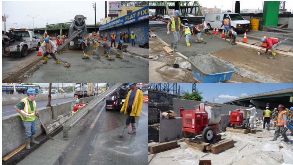
May 2012: Southbound Mainline Roadwork. June 2012: Northbound Service Road Beginning Approach.
