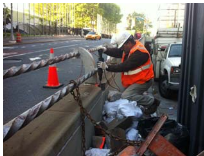
Repairing the Railing in April 2012.
