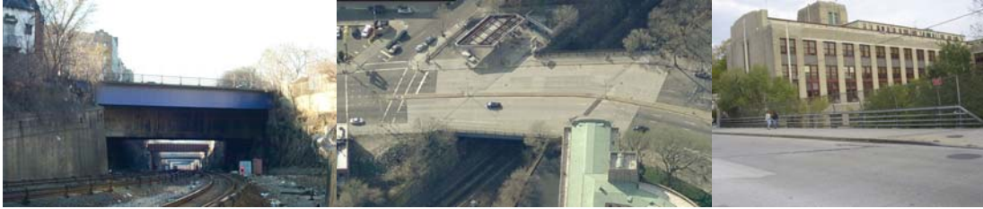
Grand Concourse Bridge over Metro North in 2002. (Credit: NYSDOT) Aerial View. Sidewalk.
