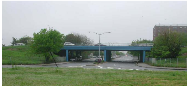
Rockaway Parkway Bridge in 2002. (Credit: NYSDOT)
