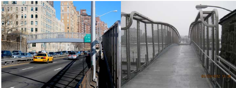
New East 78 th Street Bridge in January 2012.
