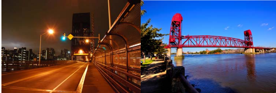
Sidewalk and Pedestrian Fence in October 2011. (Credit: Chris George and Ryan Scatenato) View of the Bridge in October 2011. (Credit: Rafael Lopez)
