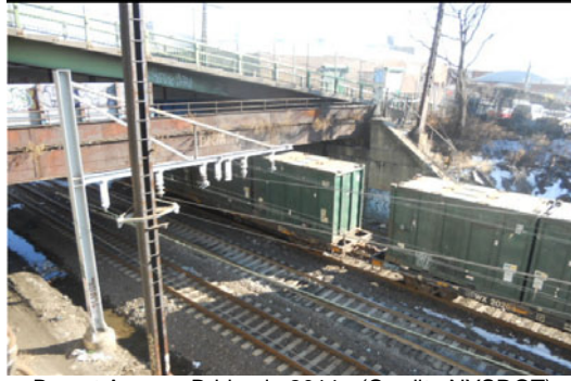
Bryant Avenue Bridge in 2011. (Credit: NYSDOT)
