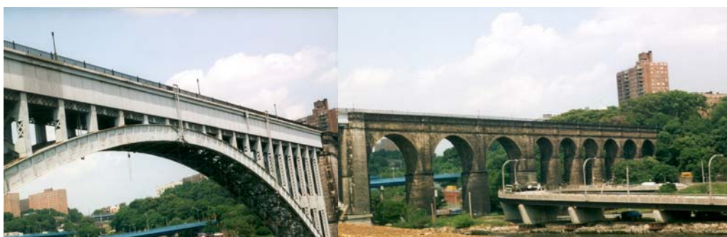
High Bridge Pedestrian Bridge in 2004. (Credit: Michele N. Vulcan)
