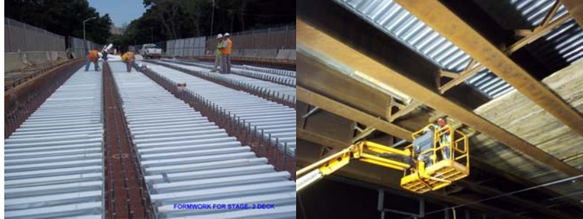
July 2012: Formwork for Stage 2 Deck. December 2012: Removing Shielding and Formwork.
