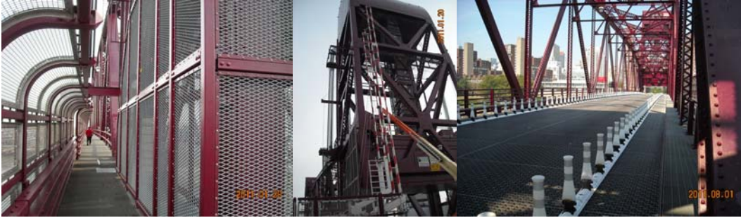
January 2011: North Sidewalk With New Pedestrian Fence. Recently Painted Bridge With New Traffic Control Equipment. View of Bridge in August 2011.
