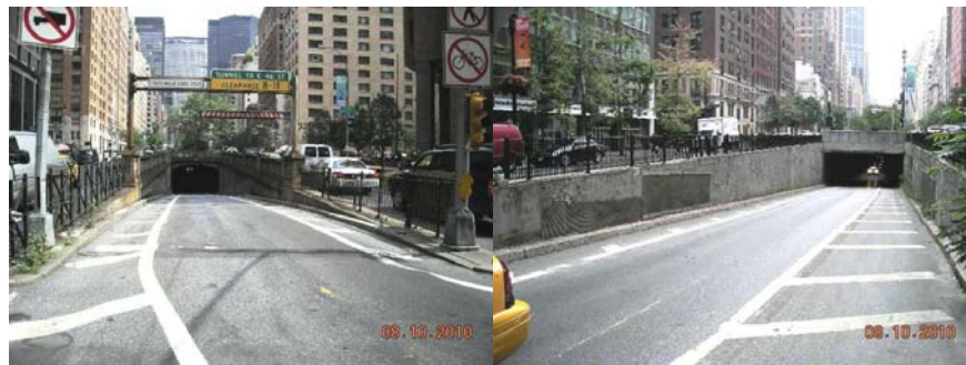
Two Views of Park Avenue Tunnel in 2010. (Credit: NYSDOT)
