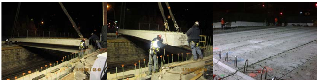
Installation of Pre-Cast Box Beams for Stage 1 in November 2011.
