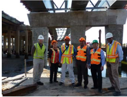
Site Visit in September 2012: Acting Director of Bridge Preventive Maintenance Paul Schwartz, Assistant Civil Engineer Evgenia Campbell, Interim Director of In-House Design Ferdinand John, and Civil Engineers Jagdish Patel, Gregory Novofastovsky, and Serge Rigaud.
