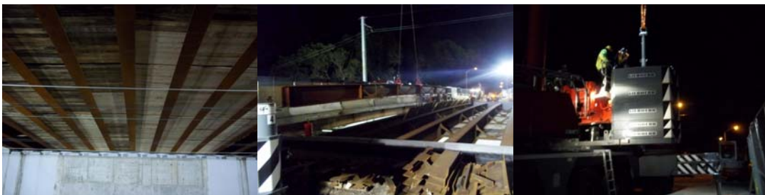
Steel Girder and Shielding Plank Installation on June 15. Disassembling the Crane.
