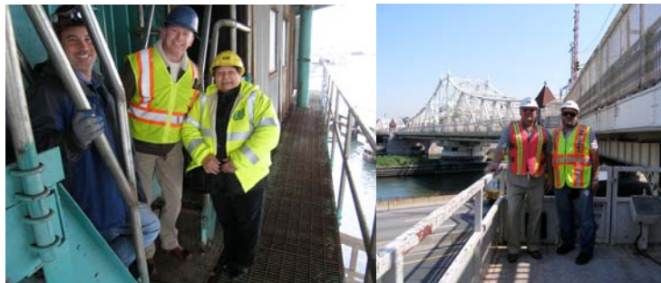
Contractor Engineer-in-Charge Scott Earl, Contractor Project Manager Tony Maracic, and Bridges Staff Analyst Antoinette Zeitoun at the Greenpoint Avenue Bridge. (Credit: Sergey Parayev) Construction Project Manager Sergey Parayev and Associate Project Manager Vadim Sokolovsky at the Macombs Dam Bridge in September 2012.
