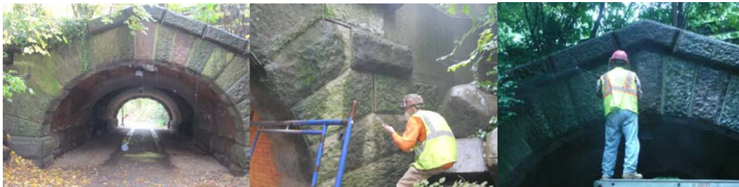
East Wood Arch. Pointing the Masonry. Cleaning the Stone Fascia.
