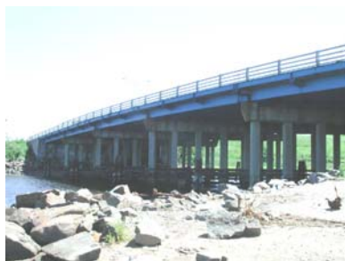
Fresh Creek Bridge in 2002. (2002 Credit: NYSDOT)
