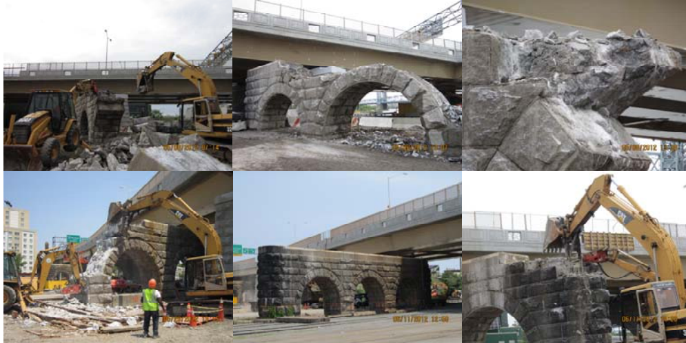
Demolition of Old Piers 13 – 15 in May and June 2012.
