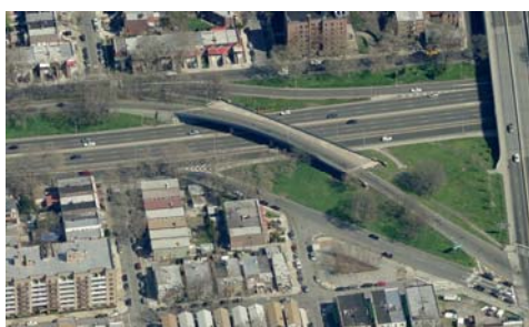
East 8 th Street Bridge Aerial View in 2009.
