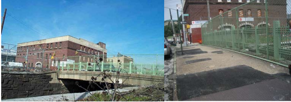
East 175 th Street Bridge in 2002. (Credit: NYSDOT) South Sidewalk.
