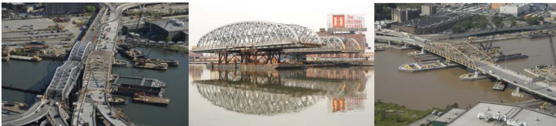
New and Old Willis Avenue Bridges on October 2, 2010. Old Willis Avenue Spans in December 2010. (Credit: Duane Bailey-Castro) Aerial View in September 2011. (Credit: Hardesty and Hanover)
