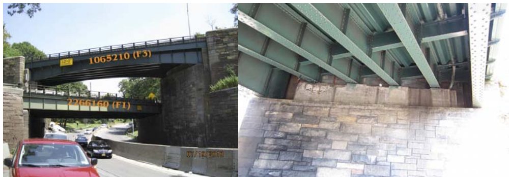
Bridge (Lower Structure) in 2010. (Credit: NYSDOT)
