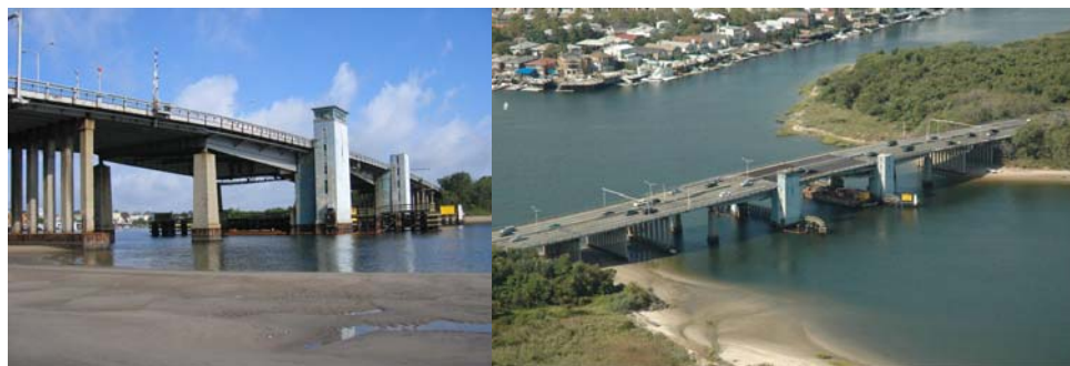
Belt Parkway Bridge Over Mill Basin. Aerial View.
