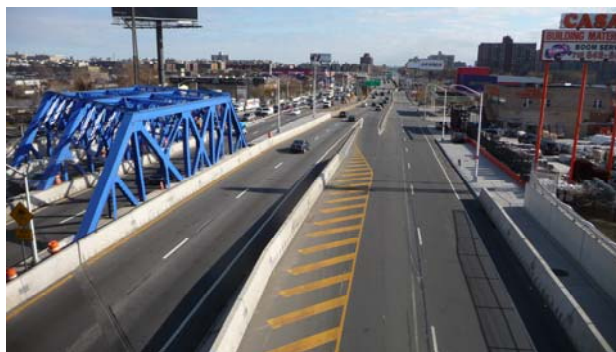
Completed Bruckner Expressway Bridges in November 2012.
