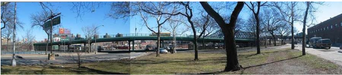
Harlem River Drive Bridge at East 127 th Street.
