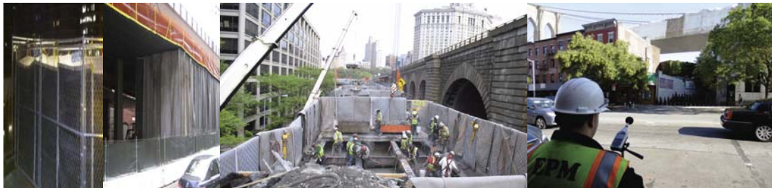
Noise Reduction Along the Sound Pathway – Acoustical Barriers on the Bridge During Night Construction Activities. Acoustical Curtains Along Frankfort Street. Two Crews Work Along Frankfort Street in April 2012. Cranes (On Left) Lift Material In And Out of Walled Enclosures of Sound Blankets. Inspector Taking Noise Measurements.
