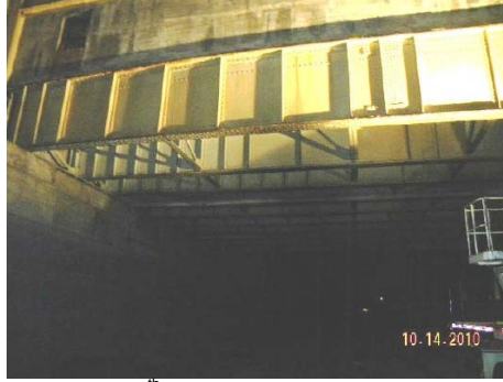
West 79 th Street Bridge Over Amtrak in 2010. (Credit: NYSDOT)
