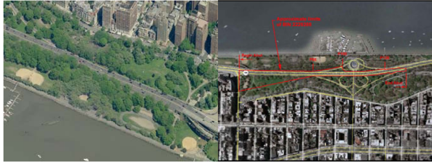
Aerial View of the Viaduct.
