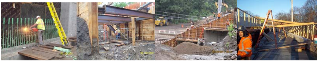
Shore Road Circle Bridge in April 2011 – July 2011. November 2011: Deck Placement.
