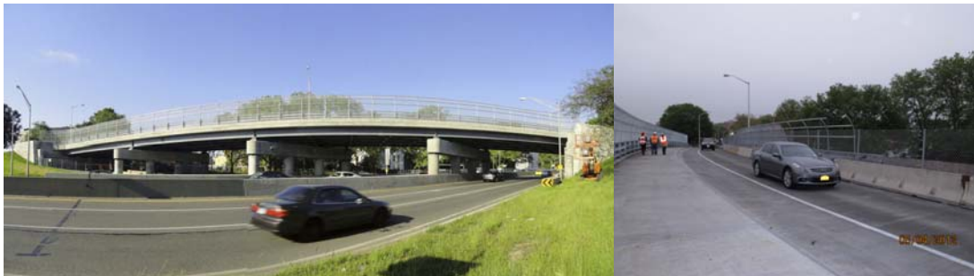
East 8 th Street Access Ramp – East Side View. Traffic on Bridge.
