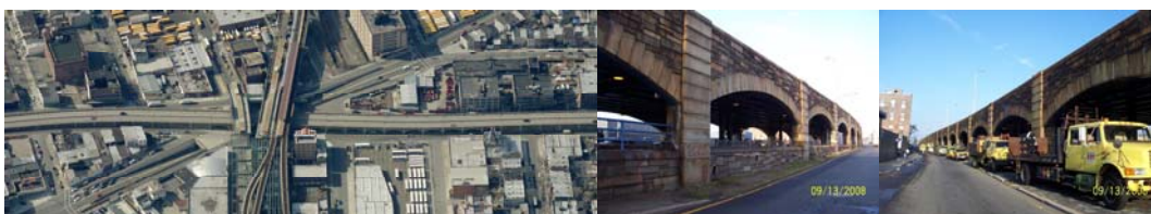
Aerial View in 2009. Elevation Left Spans 38 -43 and Elevation Right Spans 20 – 34. (Credit: NYSDOT)
