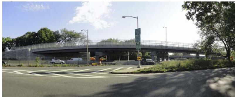
East 8 th Street Access Ramp – West Side View.
