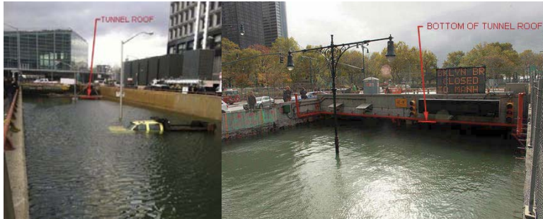
Battery Park Underpass - View Looking West at the South Portal Entrance Near the FDR Drive. View Looking South at the North Portal Entrance Near West Street. Both Tunnels Were Flooded to Their Roofs, Which Means That all Tunnel Ventilation, Electrical, and Mechanical Systems Were Entirely Submerged in Saltwater.
