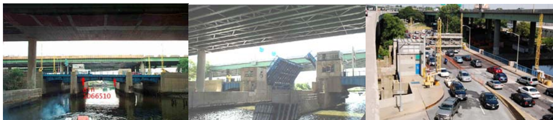
Unionport Bridge in 2002. (Credit: NYSDOT) Eastbound View.
