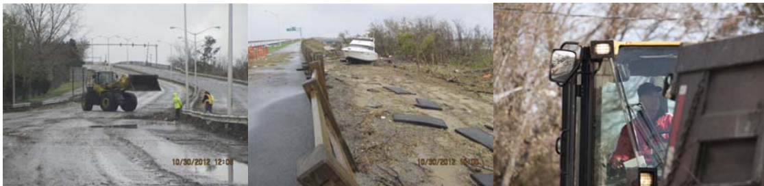
Payloader Cleaning up Debris From Hurricane Sandy on the Eastbound Belt Parkway East of Mill Basin. Private Boat Washed up on Slope of Eastbound Belt Parkway West Side of Paerdegat Basin During Hurricane Sandy. Note Damage to Bicycle/Pedestrian Path and Timber Rail. Motor Grader Operator Peter Paramithis Operating Machinery to Clear Streets in the Oakwood Beach Neighborhood of Staten Island on November 6. (Credit: Stephen Mallon)
