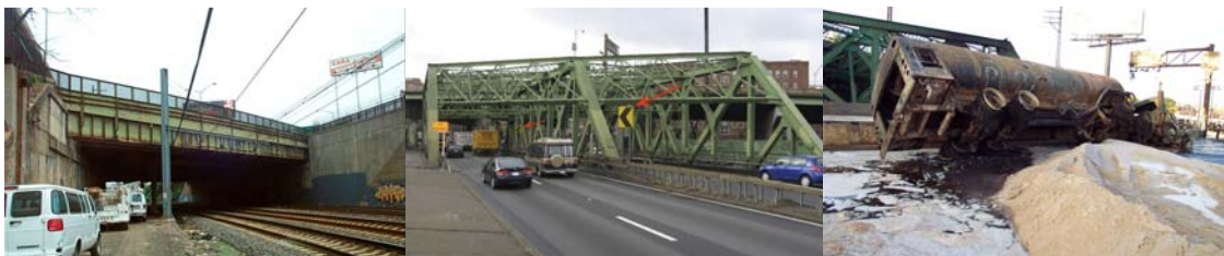
Bruckner Expressway Bridge NB in 2002. Bruckner Expressway Bridge SB in 2008. (Credit: NYSDOT) 2005: The Tanker Truck. (Credit: Bojidar Yanev)
