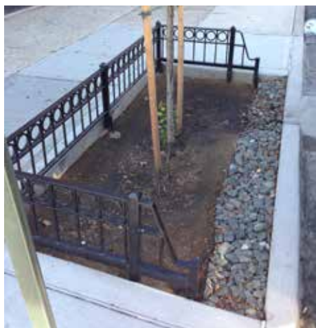
A steel tree guard is installed to protect the plants from foot traffic on the sidewalk. The tree guard posts are set in a concrete footing for stability.
