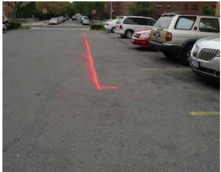
Pre-construction markout of retention/detention system
