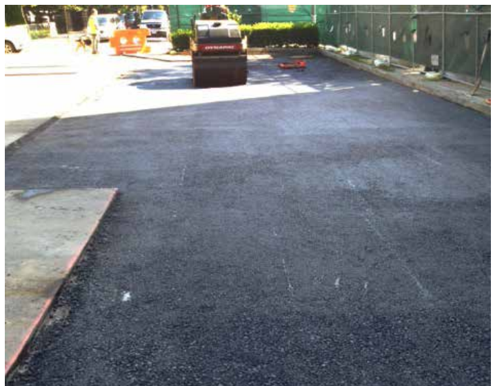
Parking lot paving restoration
