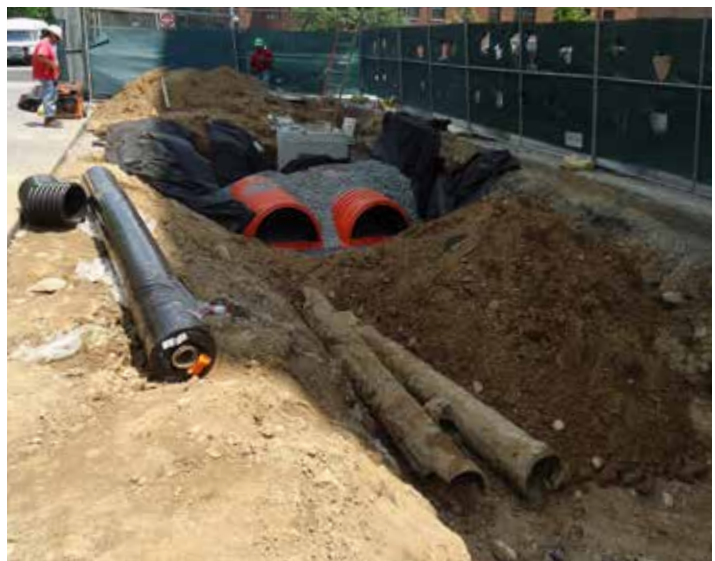
Installation of storm chambers, broken stone and new pipes
