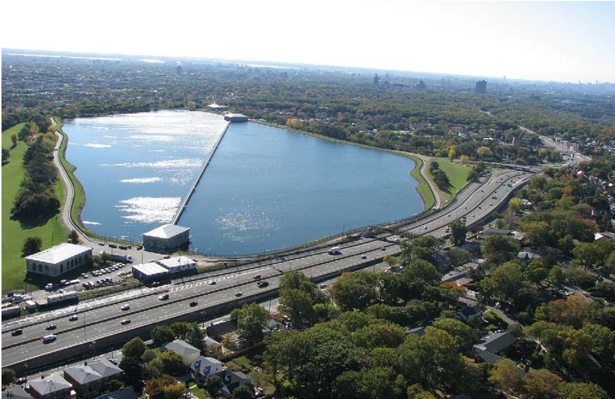
Figure 26. Hillview Reservoir aerial view of dividing wall. Photo by DEP Police.
