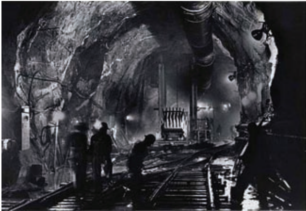
City Water Tunnel No. 3
