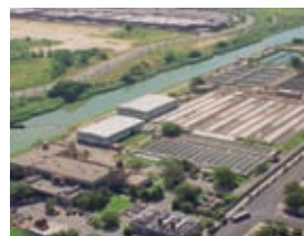
26th Ward Wastewater Treatment
