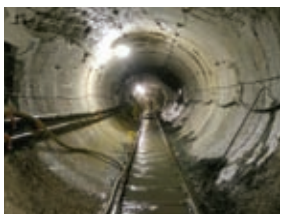
City Water Tunnel No. 3
