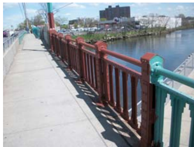
Prime Coating on East Side Hand Rails.
