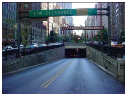
Park Avenue Tunnel in 2003. (Credit: NYSDOT)
