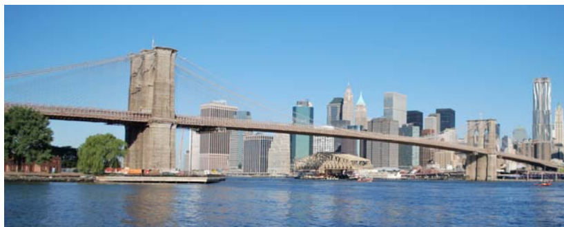
Voyage up the East River on July 26, 2010. New Willis Avenue Bridge Span Passing Under the Brooklyn Bridge. (Credit: Douglas Reese)
