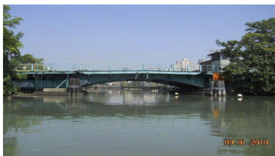
Union Street Bridge in 2010. (Credit: NYSDOT)
