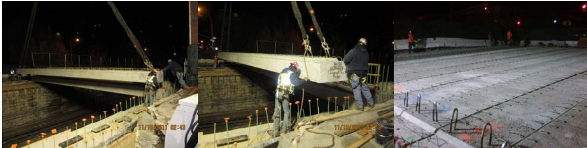
Installation of Pre-Cast Box Beams for Stage 1 in November 2011.
