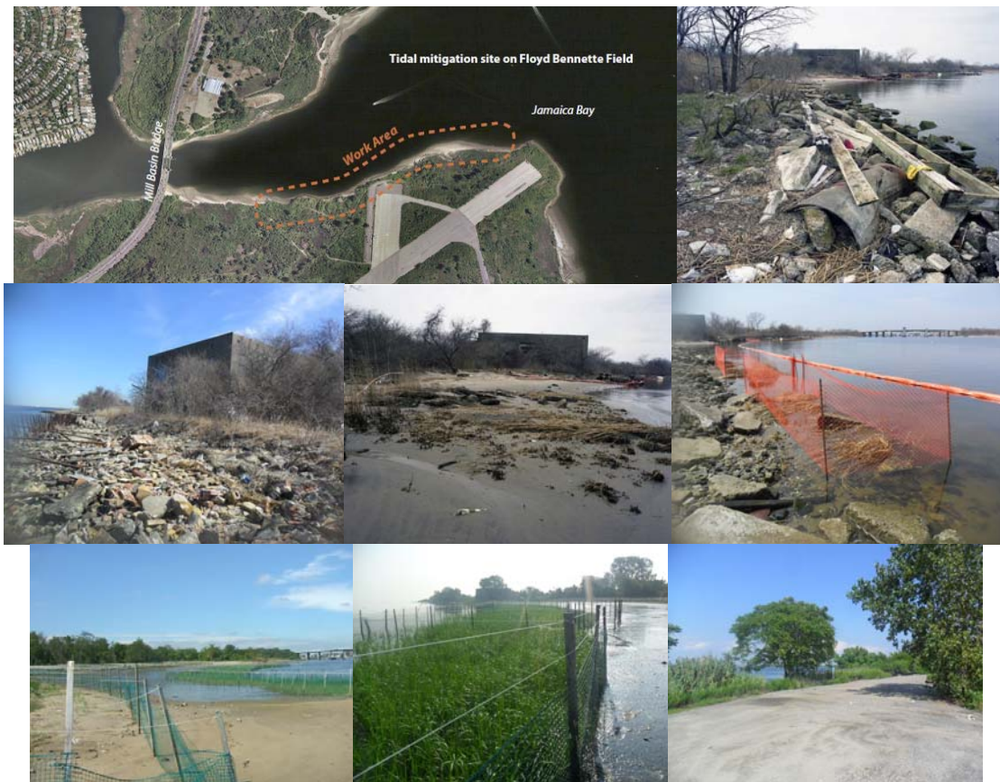
Tidal Wetland Mitigation Site. Looking West Towards Mill Basin Bridge – Shoreline Prior to and Post Cleanup. Turbidity Curtain Along Shoreline in Spring 2011. Summer and Fall 2011: Planted Wetland Grasses and Completed Uplands Planting.
