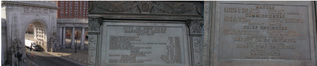
Manhattan Bridge Arch and Part of the Colonnades in March 2011. (Credit: Bojidar Yanev) Construction Plaque. (Credit: Jagtar Khinda)
