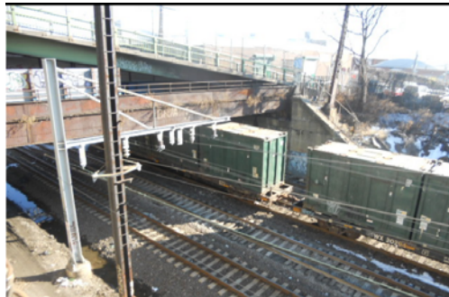
Bryant Avenue Bridge in 2011. (Credit: NYSDOT)
