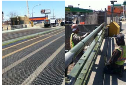
Painted Median Curb. Painting the Handrails.
