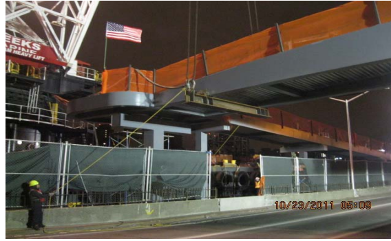
New Main Span Steel Erection in October 2011.
