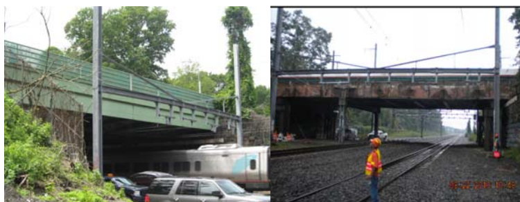
Shore Road Circle Bridge in June 2009 and August 2010. (Credit: NYSDOT)
