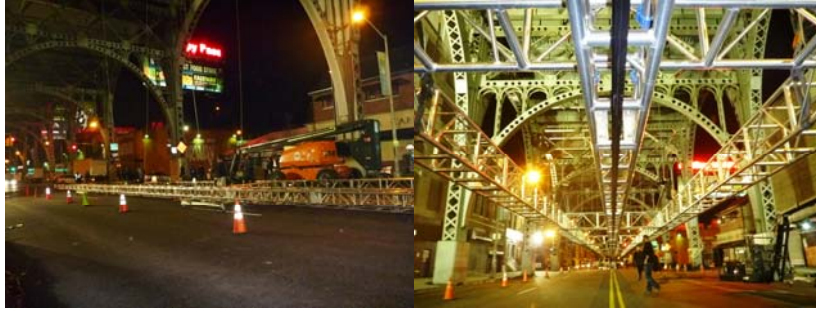
Trusses Attached to the Riverside Drive Viaduct for the Film Shoot.
