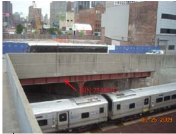
West 33 rd Street Bridge in 2009. (Credit: NYSDOT)
