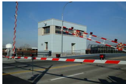
Metropolitan Avenue Bridge over English Kills Operator House.
