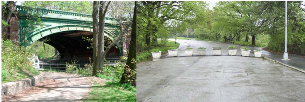
Hill Drive Bridge in 2001. Near End Approach in May 2009: Concrete Flower Pots Close the Roadway. (Credit: NYSDOT)
