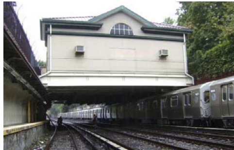
Beverly Road Bridge in 2009. (Credit: NYSDOT)
