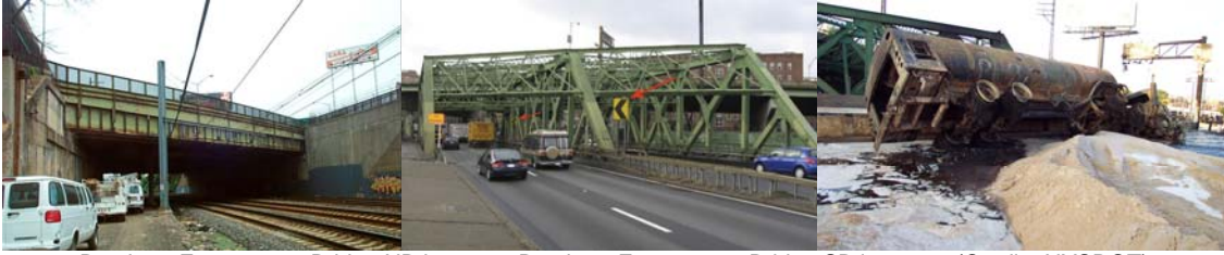
Bruckner Expressway Bridge NB in 2002. Bruckner Expressway Bridge SB in 2008. (Credit: NYSDOT) 2005: The Tanker Truck. (Credit: Bojidar Yanev)
