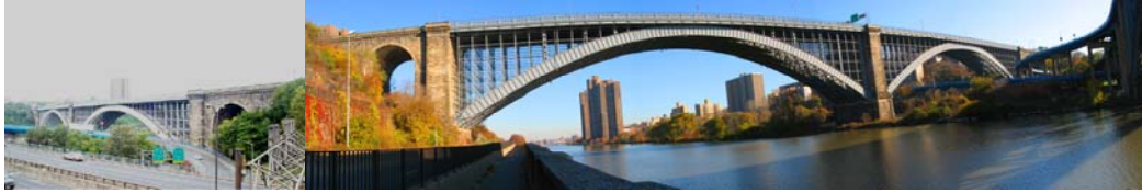
Washington Bridge. (Credit: NYSDOT) Washington Bridge in 2008. (Credit: Duane Bailey-Castro)
