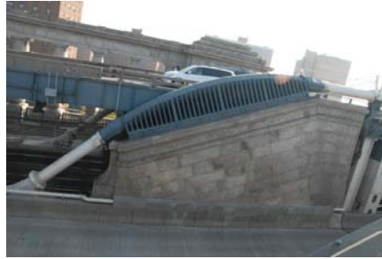
Manhattan Bridge Saddle. (Credit: Jagtar Khinda)
