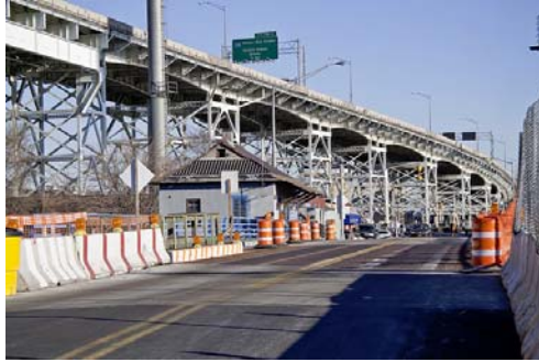
Late December 2010: Bridge Open to Vehicular Traffic. (Credit: Mitch Waxman)
