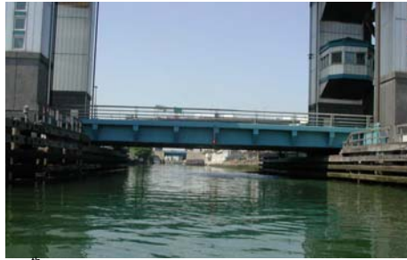
9 th Street Bridge in 2009. (Credit: NYSDOT)
