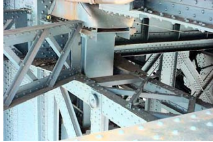
Truss Bearing on Manhattan Bridge. (Credit: NYSDOT)
