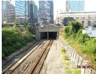
11 th Avenue Bridge in 2010. (Credit: NYSDOT)
