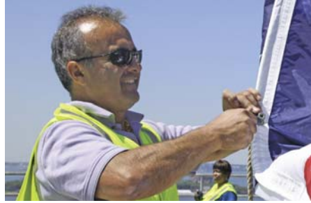
Supervisor Bridge Painter Cesar Pazmino Preparing to Hoist the Brooklyn Bridge Flag.
