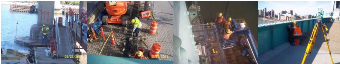
Construction in August, October, and December 2011. Installing Handrails Between Spans 7 and 9.
