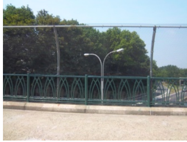
Painted Hand Rails on the Bridge.
