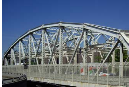
Macombs Dam Camelback Truss.
