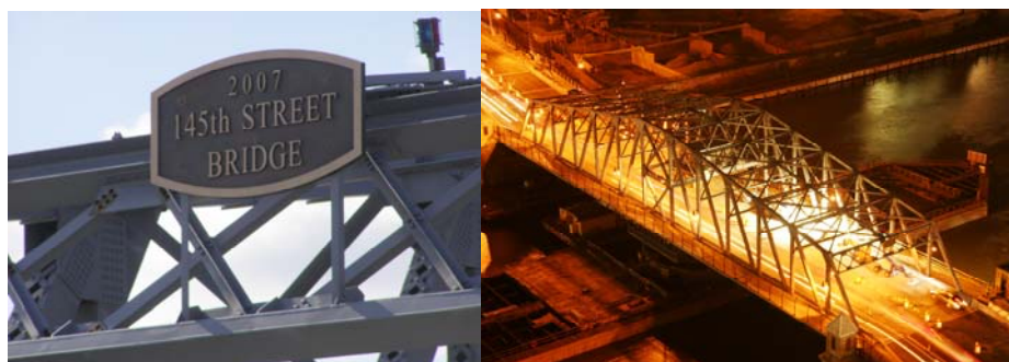
Bridge Sign. June 2007: New 145 th Bridge at Night.
