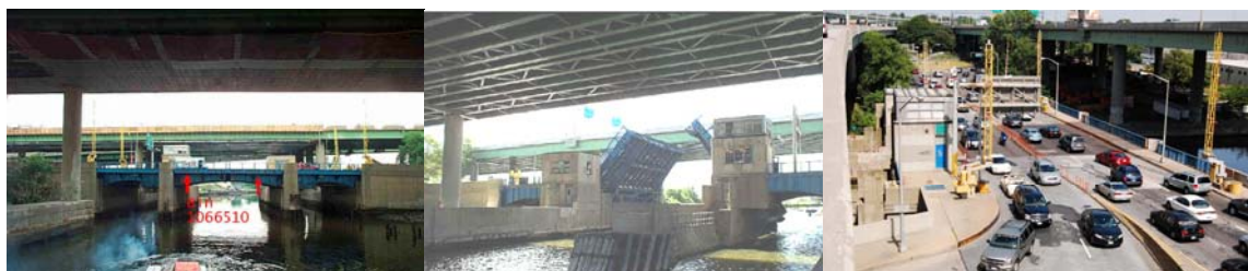
Unionport Bridge in 2002. (Credit: NYSDOT) Eastbound View.
