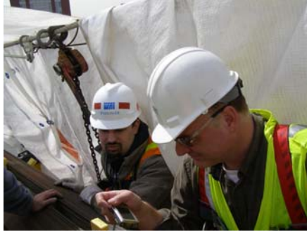
Manhattan Bridge Engineer-in-Charge Brian Gill Inspecting Cable "D."
