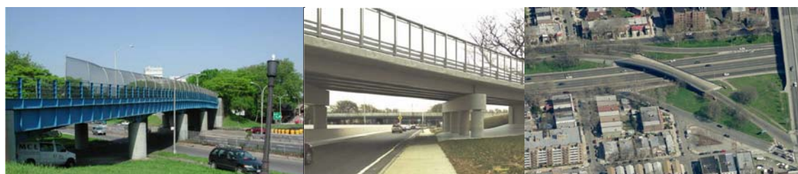
East 8 th Street Bridge in 2002. (Credit: NYSDOT) Rendering of New Bridge. Aerial View in 2009.
