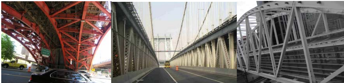
Brooklyn Bridge Franklin Square Truss. (Credit: Andy Hoang). General view of Manhattan Bridge Trusses B and C From the Lower Roadway on the Main Span. (Credit: NYSDOT) Chambers Street Pedestrian Bridge Truss.
