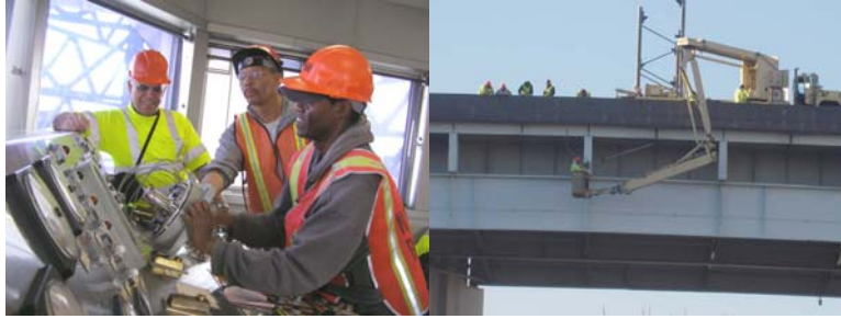
Construction Project Manager Gholamali Mozaffari, and Electricians Nelson Crooks and Gary Emmanuel Fixing Machinery in the Ninth Street Bridge Operator House in April 2008. (Credit: Vera Ovetskaya) Repairing the Navigation Lighting on the Hunterspoint Bridge. On the Bridge: Oilers Carl Wharton, Richard Morreale, and Paul Califano, Mozaffari Ali, Electrician Naum Golburt, and Highway Repairers Manny Nardiello and Kevin Donahue. In the Snooper Bucket: Harry Parmaman and Supervisor Electrician Jose Done. (Credit: Samuel Teaw)
