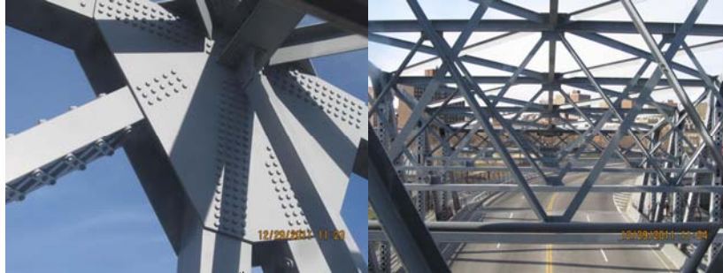
145 th Street Bridge in December 2011.
