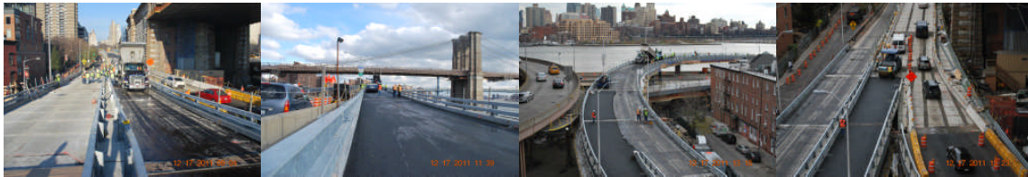
December 2011: Ramp C.
