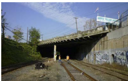
Metropolitan Avenue Bridge in 2009. (Credit: NYSDOT)
