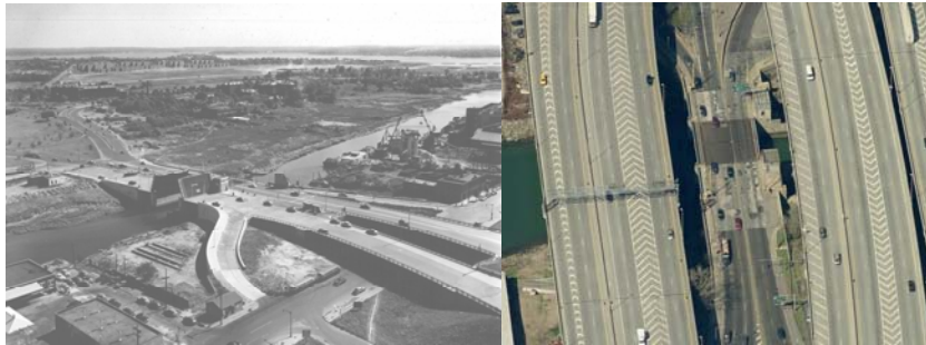
Unionport Bridge in 1953 and 2009.
