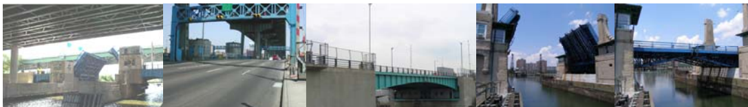
Unionport Bridge. (Credit: NYSDOT) Hamilton Avenue Bridge. (Credit: NYSDOT) Union Street Bridge. Greenpoint Avenue Bridge. (Greenpoint Credit: Michele N. Vulcan) Shore Road Bridge in July 2011. (Credit: Sergey Parayev)
