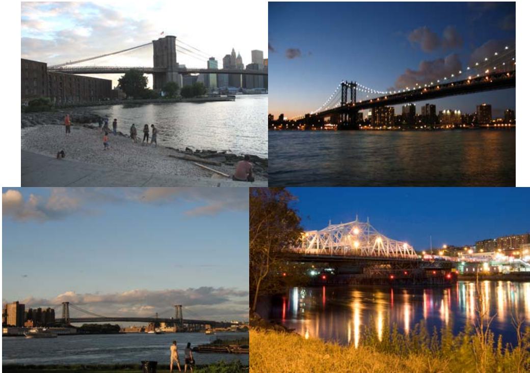
Brooklyn, Manhattan, and Williamsburg Bridges. (Credit: Michele N. Vulcan) University Heights Bridge in October 2010. (Credit: Duane Bailey-Castro)
