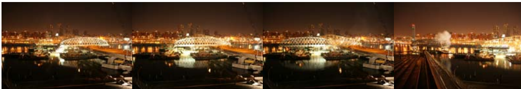
Floating Out the Flanking Span on April 12, 2011.
