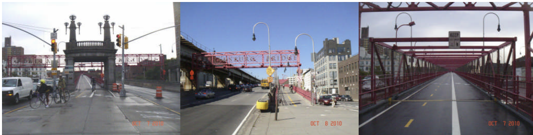
Manhattan and Brooklyn Approaches and Pedestrian Walkway in October 2010. (Credit: NYSDOT)
