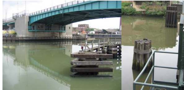
Greenpoint Avenue Dolphin & Fender System. (Credit: Peter Basich) Hunters Point Avenue Dolphins. (Credit: Michele N. Vulcan)
