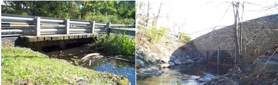
Idlease Place Culvert. Sweet Brook Road Culvert.
