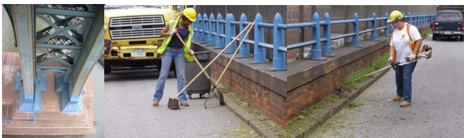
Manhattan Bridge Tower After Debris Removal. (Credit: Peter Basich) 161 st Street Pedestrian Bridge Over Major Deegan Expressway. Assistant City Highway Repairer Lashawn Elam and Highway Repairer Anita Ramos Removing Vegetation and Other Debris.
