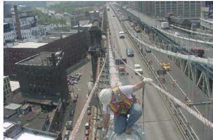
Inspector on Manhattan Bridge Cable. (Credit: NYSDOT)
