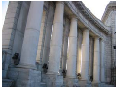
Manhattan Bridge Colonnade. (Credit: Peter Basich)
