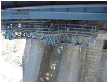
Manhattan Bridge Traveler. (Credit: NYSDOT)
