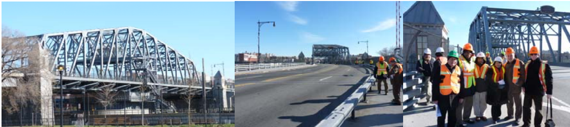
Civil Engineers Ferdinand John and Edvard Jeamgocian Examining the Sidewalk. (Span and Sidewalk Credit: Alexander Berens) At the Walk-Through Inspection on December 29, 2011: Civil Engineers Gregory Novofastovsky and Ferdinand John, Director of Quality Assurance Engineer Muhammad Afzal, Civil Engineers Svetlana Kaganovskaya and Edvard Jeamgocian, and Assistant Civil Engineer Alexander Berens.
