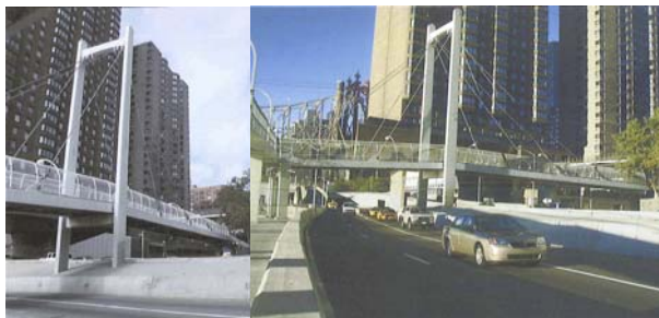
East 64 th Street Pedestrian Bridge over FDR Drive.
