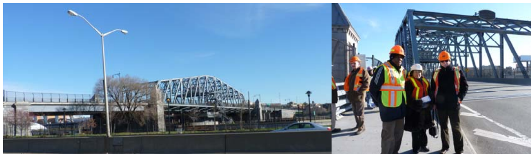
145 th Street Bridge. (Credit: Alexander Berens) Civil Engineers Ferdinand John and Svetlana Kaganovskaya, and Assistant Civil Engineer Alexander Berens at the Walk-Through Inspection on December 29, 2011.
