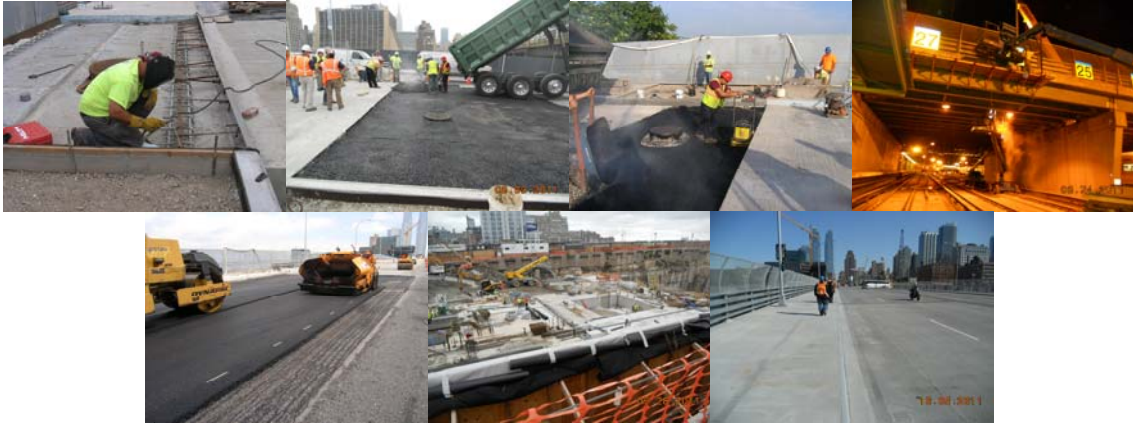
11 th Avenue Viaduct Construction in June 2011. August 2011. September and October 2011.
