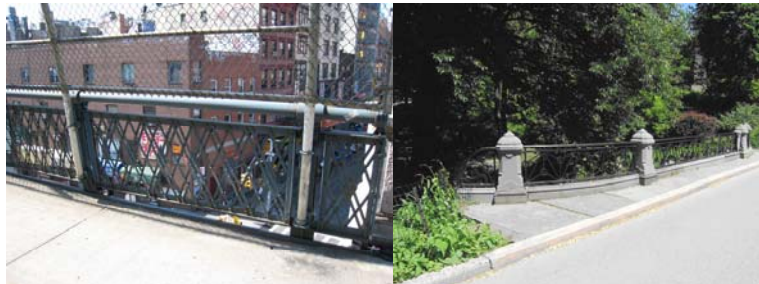
Manhattan Bridge Railing. (Credit: Russell Holcomb) Greywacke Arch Railing.
