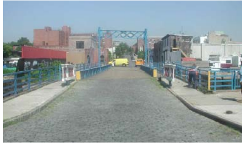
Carroll Street Bridge Approach. (Credit: NYSDOT)
