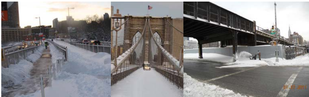
Inspecting and Clearing the Brooklyn Bridge Walkway on January 27. (Credit: Hayes Lord) Clearing Snow at the 11 th Avenue Viaduct Project.
