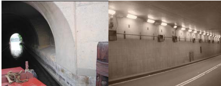
Hamilton Avenue Bridge and Battery Place Underpass Abutments. (Credit: NYSDOT)
