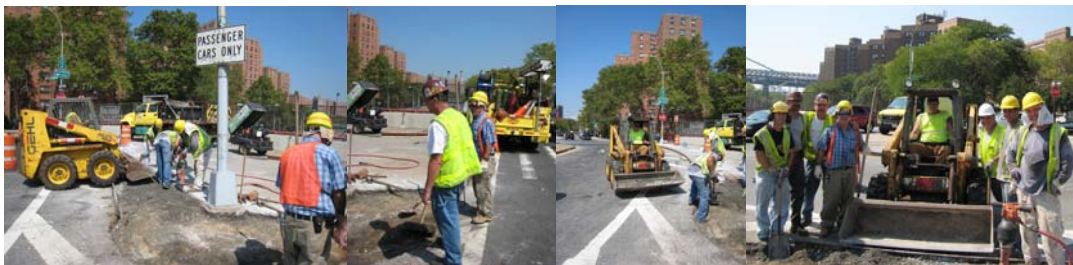
Sidewalk Repairs in August 2010 at Houston Street Bridge over the FDR Drive: Tractor Operator Robert Noordzy (in Tractor), Bricklayer Vincent Sciulla, Cement Masons Frank Finizio and Victor Porowski, and Bricklayer Luigi Cuffari. Bridge Repairer and Riveter Brook Budd and Bricklayer Luigi Cuffari. Tractor Operator Noordzy (in Tractor), Cement Masons Frank Finizio (Foreground) and Victor Porowski (Background), and Bricklayer Vincent Sciulla. Bricklayer Vincent Sciulla, Bridge Repairer and Riveters James Philip and Brook Budd, Bricklayer Luigi Cuffari, Tractor Operator Robert Noordzy, Supervisor Bricklayer Edward Alfano, and Cement Masons Frank Finizio and Victor Porowski. (Credit: Russell Holcomb)
