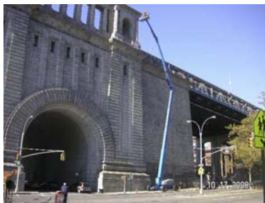
Inspecting the Exterior of the Manhattan Bridge Anchorage. (Credit: NYSDOT)
