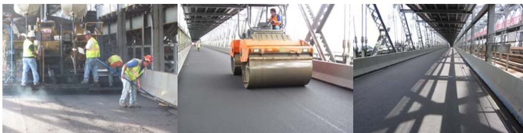
Repaving the Williamsburg Bridge in 2011.
