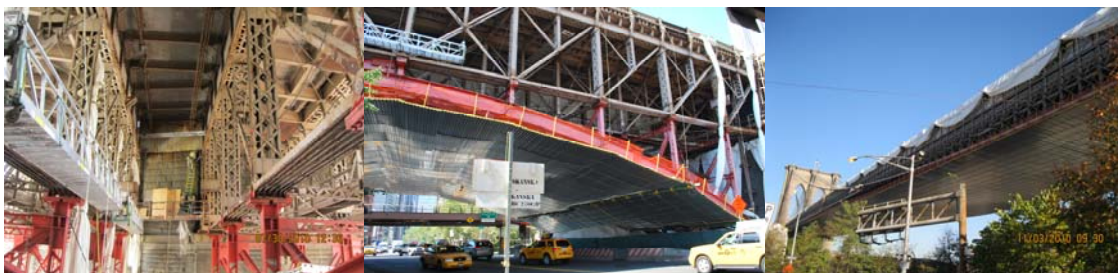
Assembly of Containment System at Franklin Square – in July and September 2010. Brooklyn Bridge Side Span Containment System – in November 2010.
