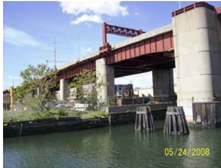
Pulaski Bridge in 2008. (Credit: NYSDOT)
