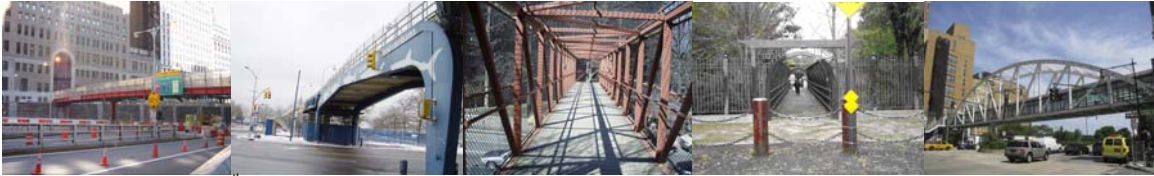
Morris Street, West 8 th Street, PS-5, Carroll Street over Franklin Shuttle, and Chambers Street Pedestrian Bridges.
