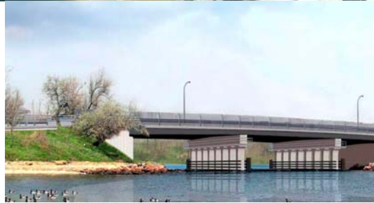
Fresh Creek Bridge Aerial View and in 2002. (2002 Credit: NYSDOT) Proposed Fresh Creek Bridge.
