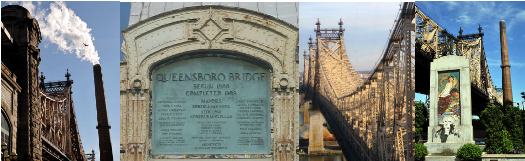
Ed Koch Queensboro Bridge in 2009. (Credit: Bernard Ente) Close-up of the 1909 Dedication Plaque. (Credit: Peter Basich) Bridge in February 2011. (Credit: Brian Gill) The Granite Fountain, Built in 1918 for a Farmers' Market Beneath the Bridge, was Rededicated in June 2003 After Restoration. Evangeline Blashfield was the Model for the Fountain's Glass Mosaic of a Woman With a Cornucopia. Her Husband, Artist Edwin Blashfield, Designed the Work. (Description: Greater Astoria Historical Society, Roosevelt Island Historical Society. Credit: Bernard Ente)
