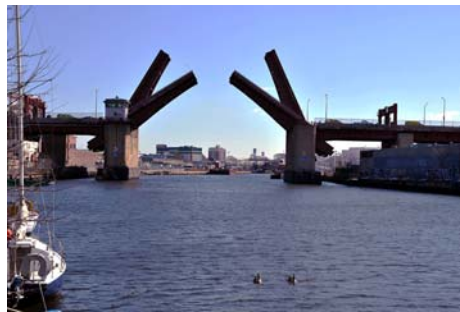
Pulaski Bridge Opening in February 2010. (Credit: Bernard Ente)
