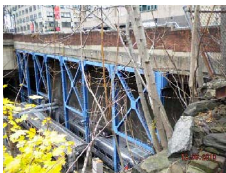
West 31 st Street Bridge in 2010. (Credit: NYSDOT)
