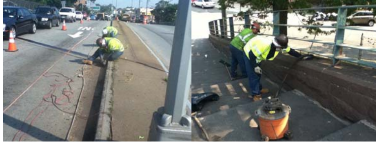
Cleaning and Painting the Hand Rails and Sidewalk Curb.
