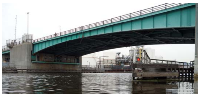
Greenpoint Avenue Bridge in April 2011. (Credit: Sergey Parayev)
