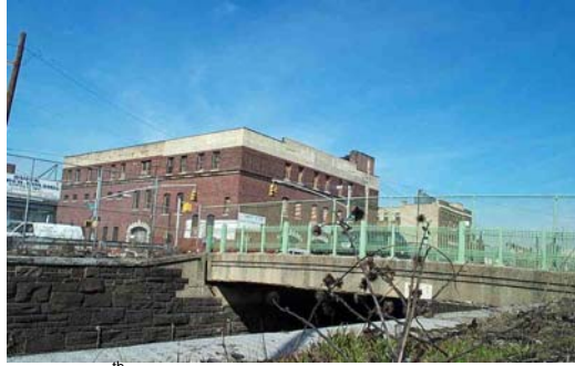
East 175 th Street Bridge in 2002. (Credit: NYSDOT)
