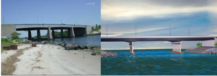
Gerritsen Inlet Bridge in 2002. (Credit: NYSDOT) Proposed Gerritsen Inlet Bridge.
