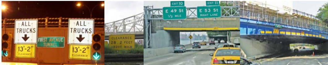
United Nations – 1 st Avenue Tunnel and Macombs Dam Bridge Vertical Clearance Postings. (Credit: NYSDOT) Retro-reflective Material Improves Visibility of These Low Vertical Clearance Bridges: East 60 th Street Bridge Over FDR Drive and Westchester Avenue Bridge over Hutchinson River Parkway.
