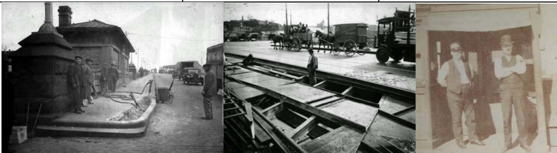
Willis Avenue Bridge Curbing and Road Repair in the Early 1920's. Gateman J. J. McDonough (on left), Great-Grandfather of Deputy Chief Engineer Russell Holcomb
