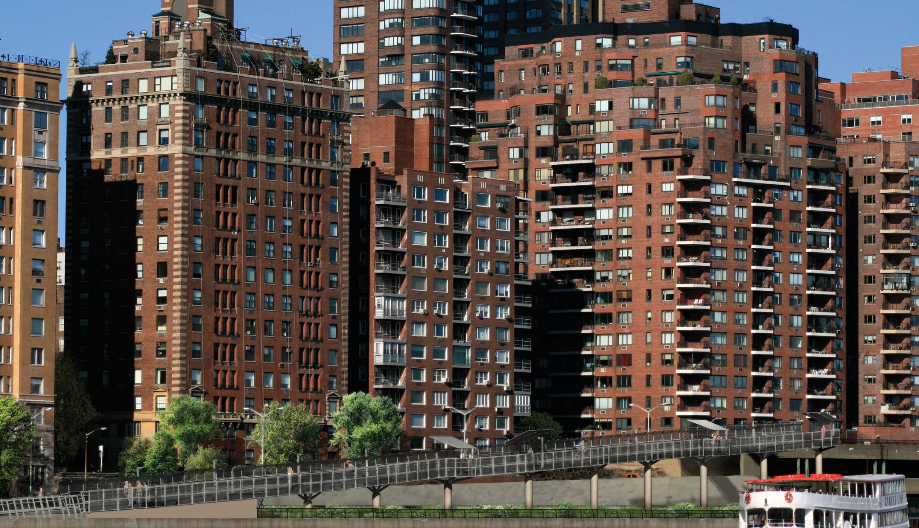
E. 81st Street Pedestrian Bridge
