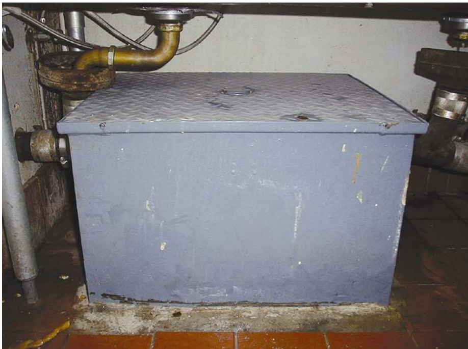
Image 3.2—Grease traps are small installed devices that remove grease from a sink's wastewater.
