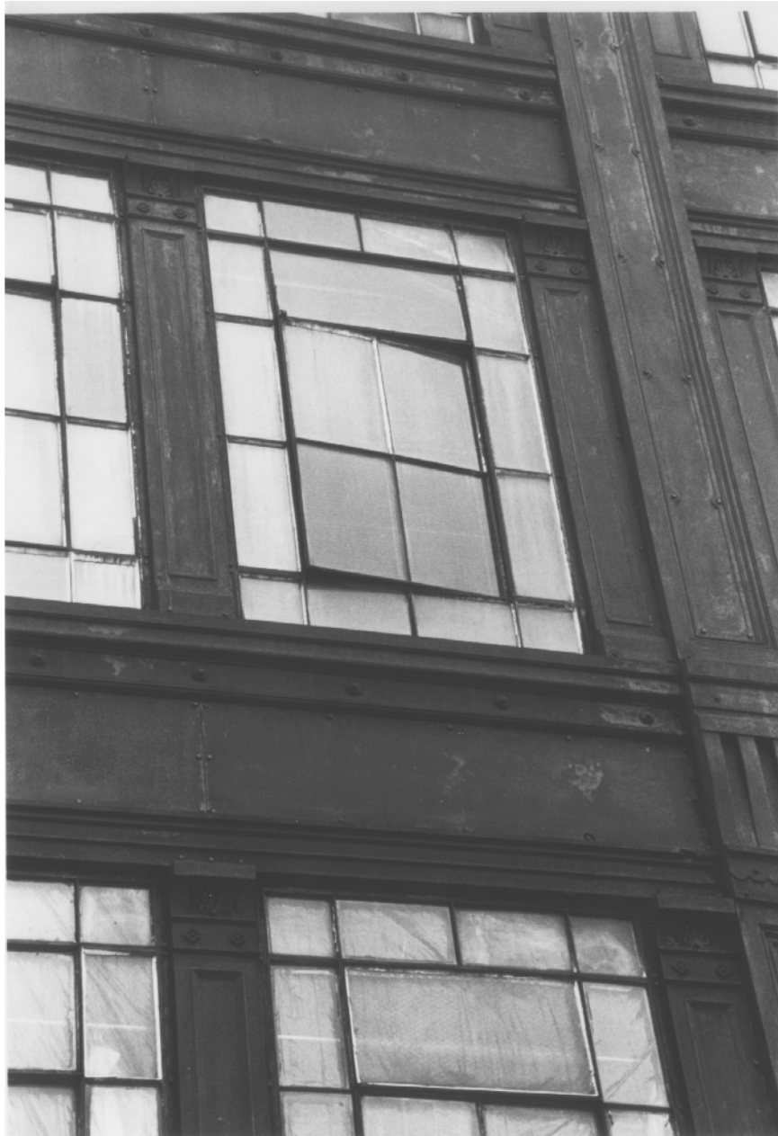
Hecla Iron Works Building Windows and pilasters Photo: Carl Forster
