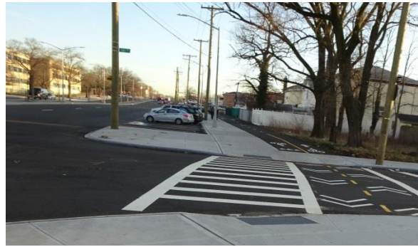
Springfield Blvd After reconstruction
