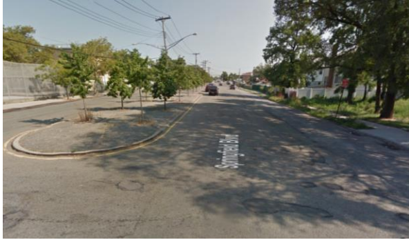
Springfield Blvd Before reconstruction
