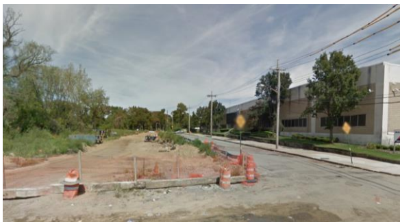
Springfield Blvd Before reconstruction
