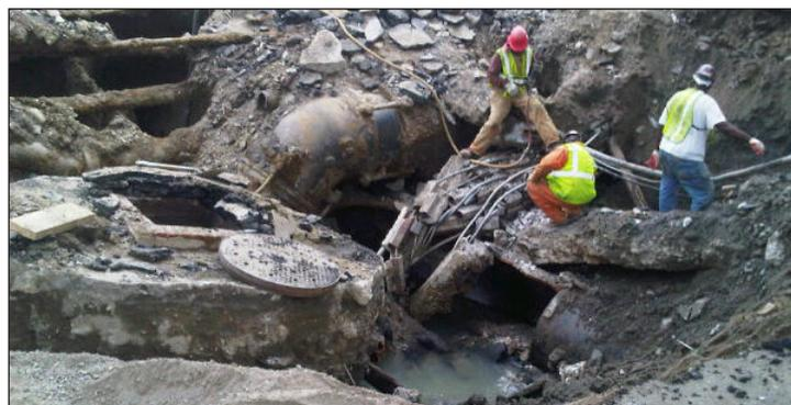
**REPAIR AND RESTORE:** Site of Jerome Avenue 36-inch water main break after the water was pumped out. Beneath New York City streets is a maze of water, sewer, electrical and gas pipes.
