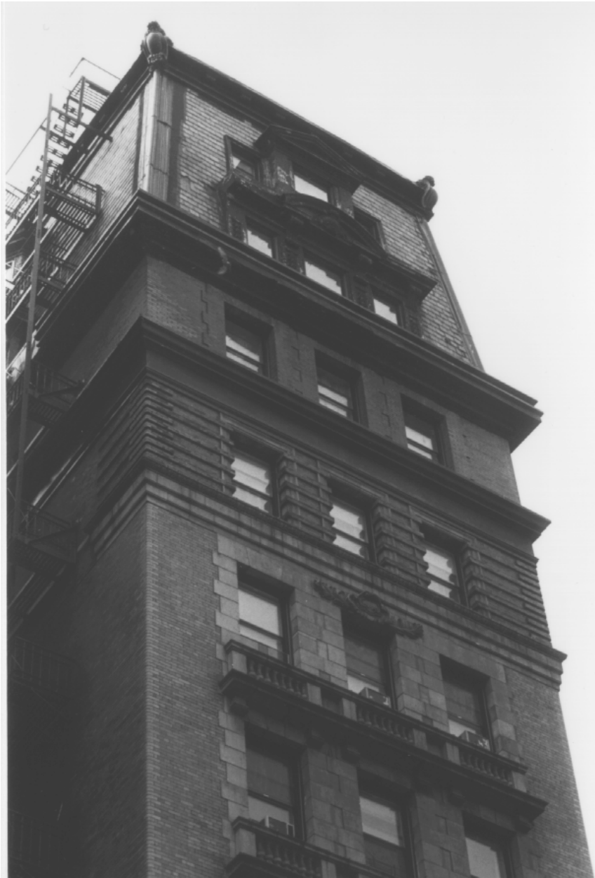
Detail of mansard roof—West 108th Street wing Photo: Carl Forster, 1996
