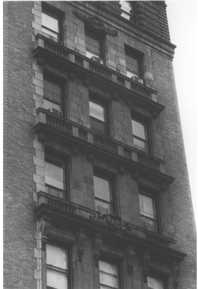
Detail of windows—5th to 7th floors Photo: Carl Forster, 1996
