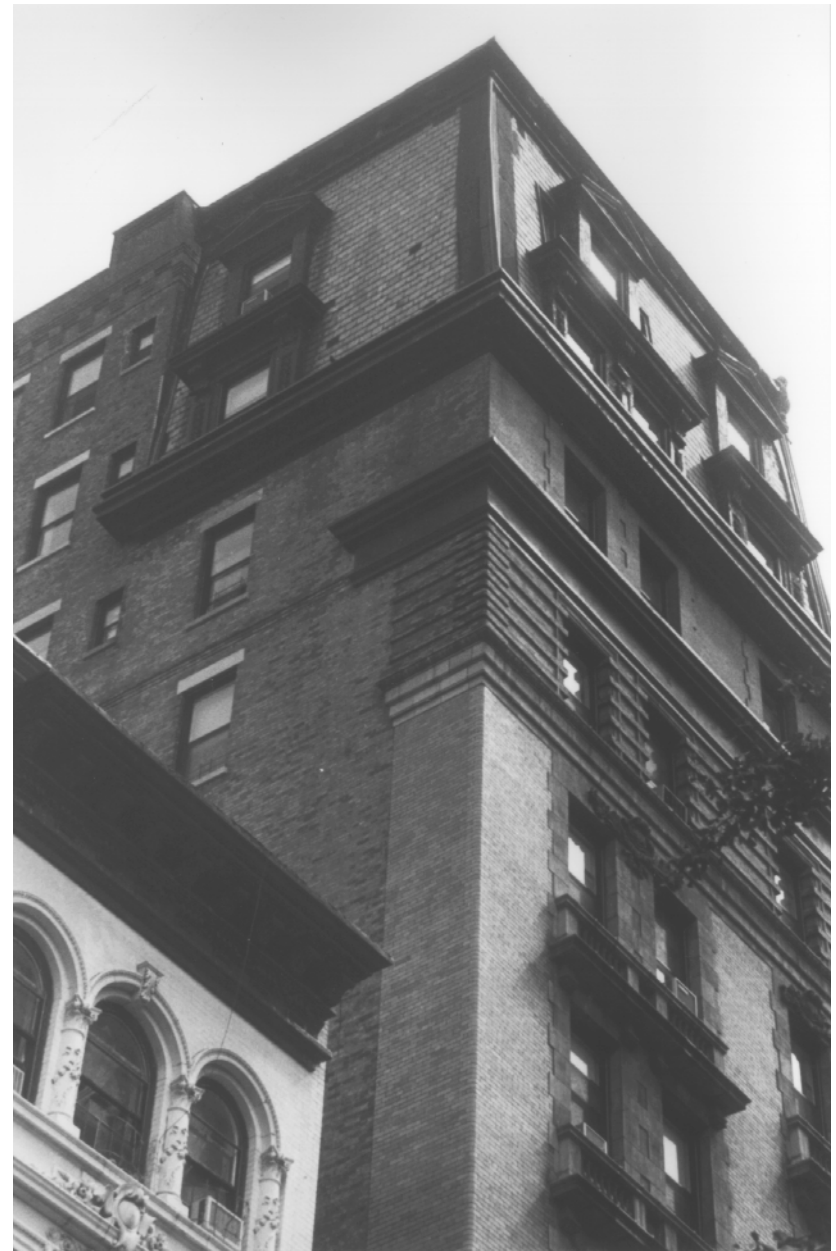
Detail of west elevation at roof level Photo: Carl Forster, 1996
