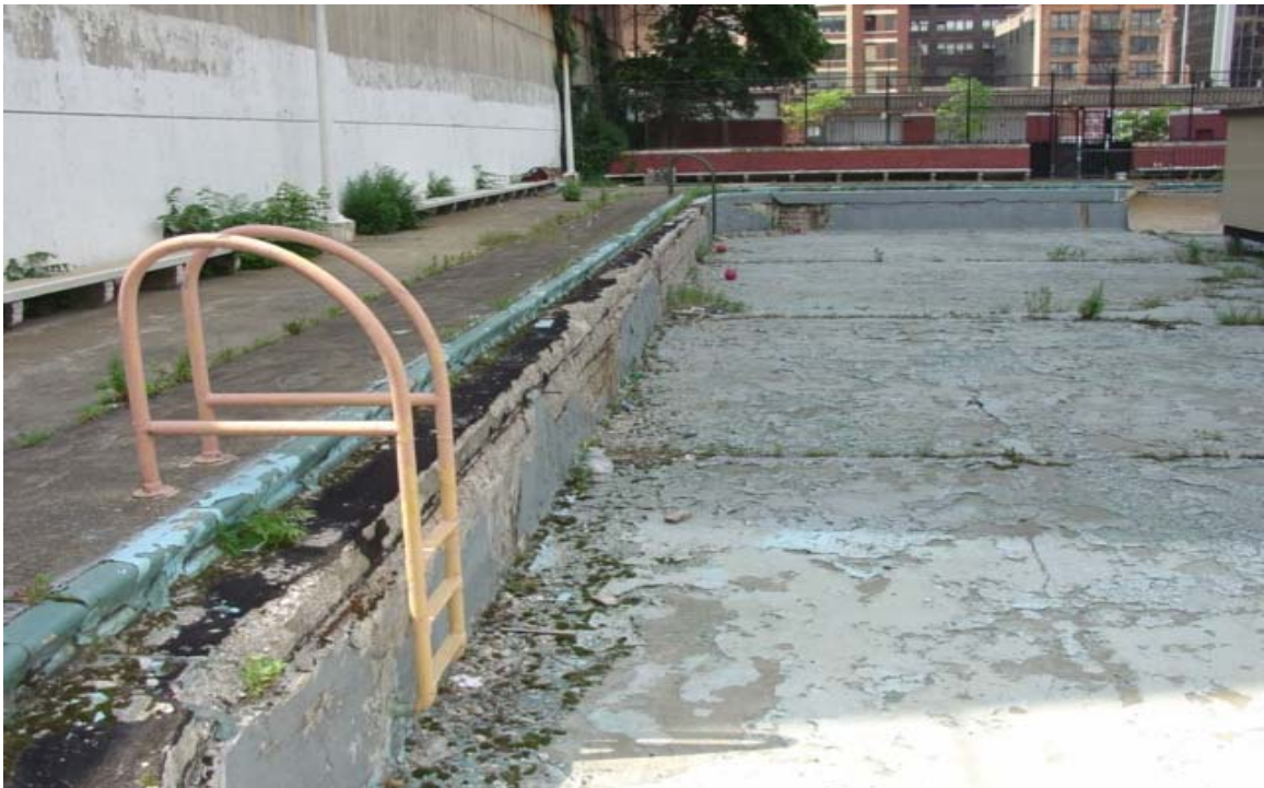
Picture #2 – Weeds and cracked flooring of outdoor swimming pool
