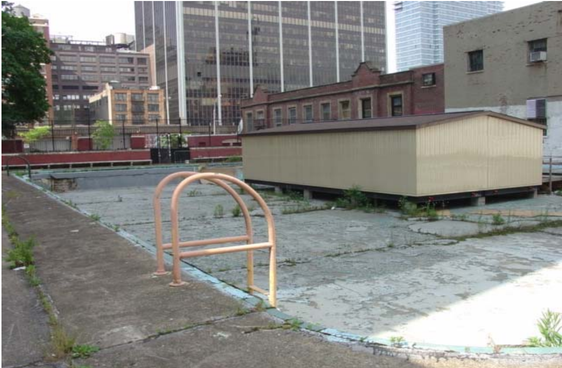
Picture #2 – Weeds and cracked flooring of outdoor swimming pool
