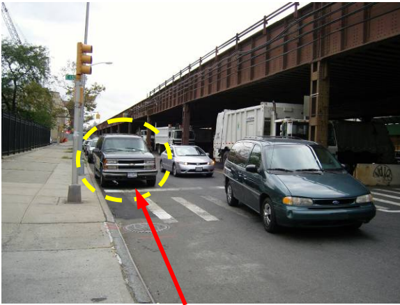
Park Avenue NB at E 132 nd Street, looking south
