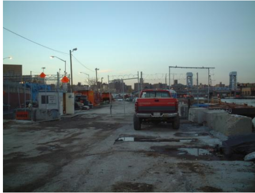
Construction staging area at waterfront
