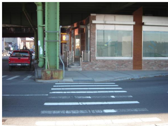
Marginal St and 125 th St: With new pedestrian traffic signal, crosswalk and curb cut
