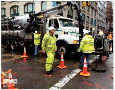
ast Friday, DEP emergency crews responded to a broken water main under 5<sup>th</sup> Avenue at 12<sup>th</sup> Street in Manhattan. The 30-inch main was originally installed in 1908. Crews continue to work to carefully repair the main. Because of their methodical approach to the repair, not one customer has experienced a disruption to their water service.
