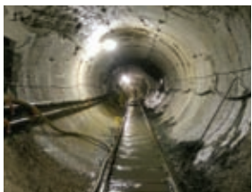
City Water Tunnel No. 3
