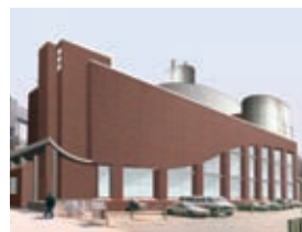
Manhattan Pumping Station
