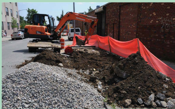
Right-of-way Bioswale construction, Junius St. and Liberty Ave., Brooklyn
