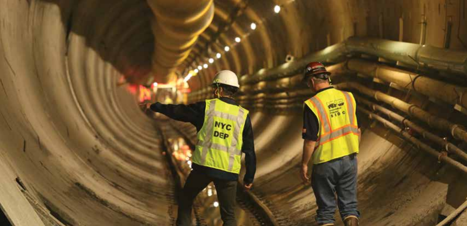
Delaware Aqueduct Bypass Tunnel
